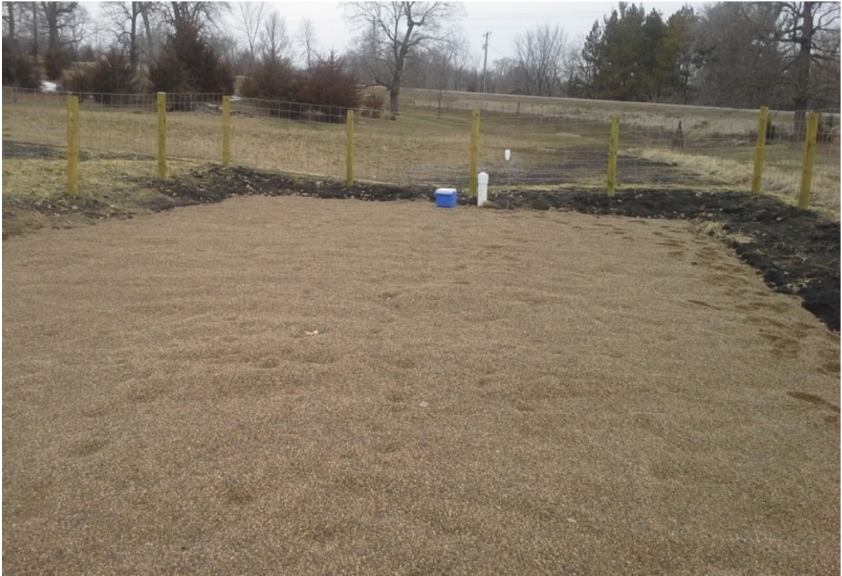
Figure 17. Site photo of Iron Enhanced Sand Filter (IESF) shortly after construction.
