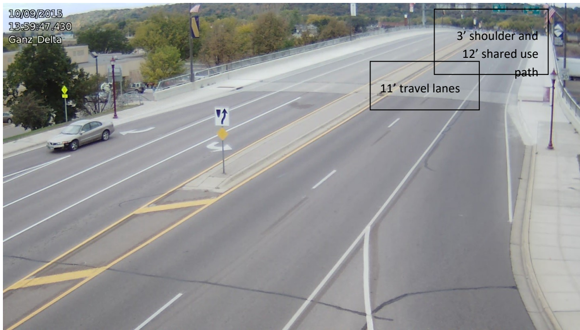
Figure 4.2 Mankato Study Site: Post-Construction
