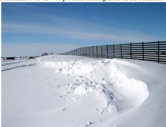
Figure 6-4. Structural Snow Fence
