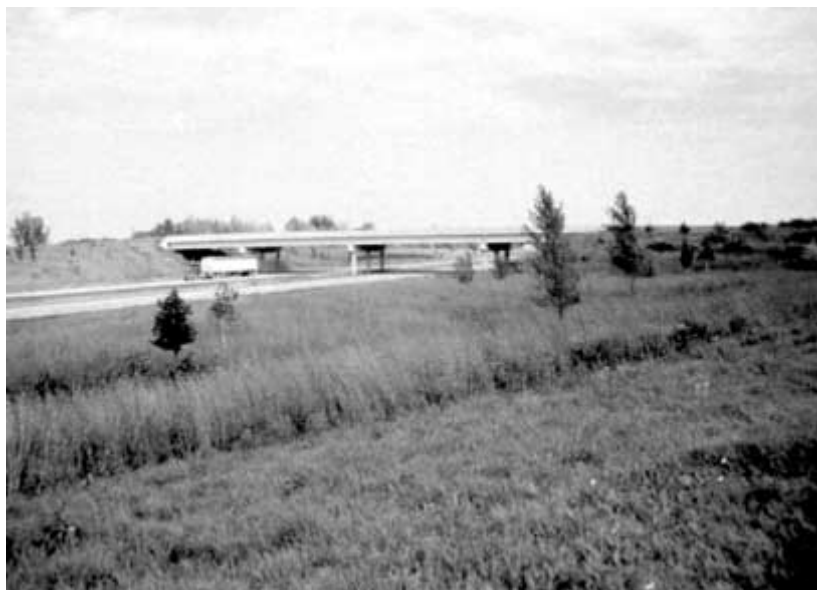
Prairie Restoration Project on Interstate 90
