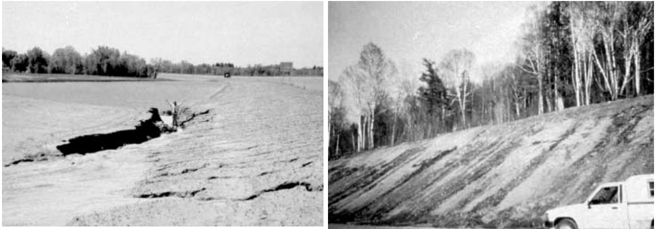
Figure B-2. Significant erosion problems can occur during construction before new turf is established
