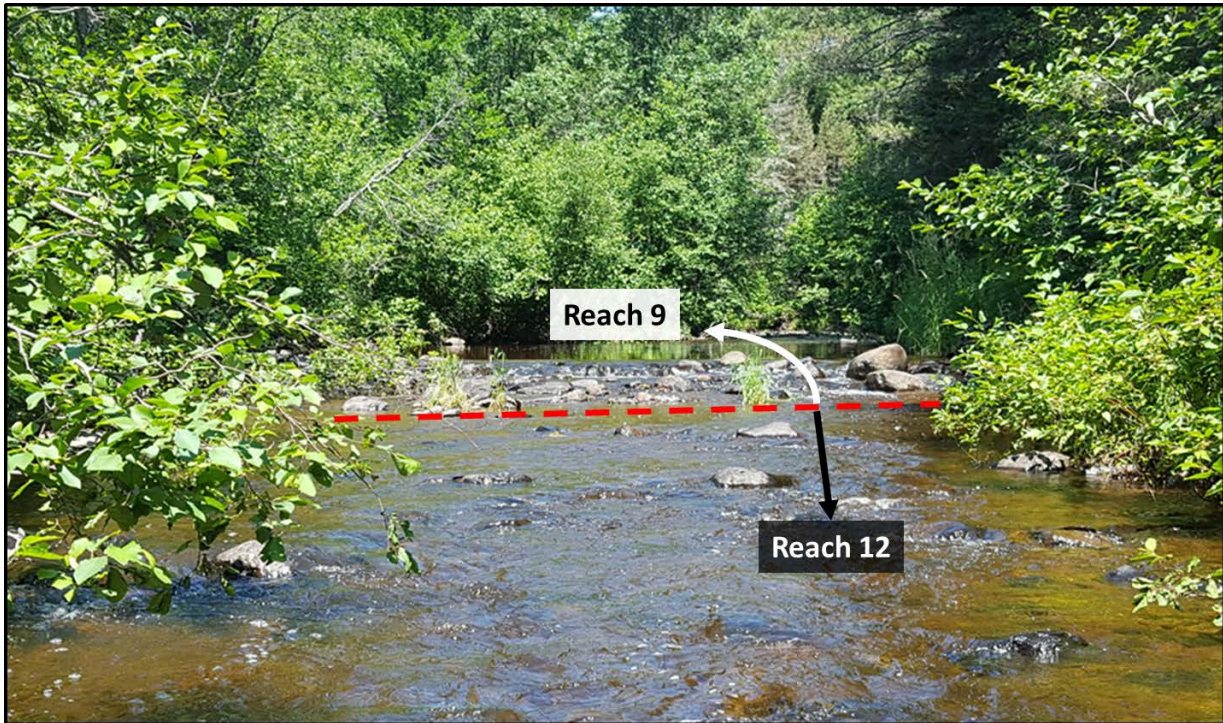
Figure 3. Photo showing the rock riffle grade-control that marks the end of Reach 12 and the beginning of Reach 9.
