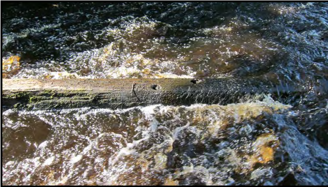
Figure 20: Cribwork timber at Site 21PN096 with peg holes affixed to the middle of the streambed on the Lower Tamarack River. (May 2013)
