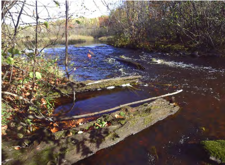
Figure 62. Color quick view of the Tamarack Creek Dam (21PN096), looking east. The image shows log ruins of the sluiceway.
