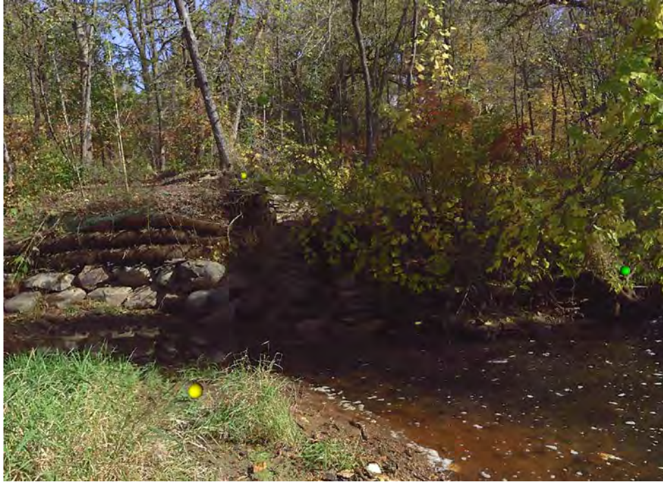
Figure 60. Color quick view of the Godfrey Dam, looking southeast.
