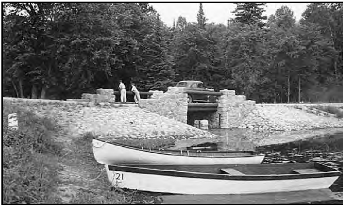
Figure 10: CCC/WPA dam/bridge built at Elk Lake in Itasca State Park. Note rusticated abutments and piers added to the typical Type “C” stop-log slots. (MHS collections photo SD11t r7)
