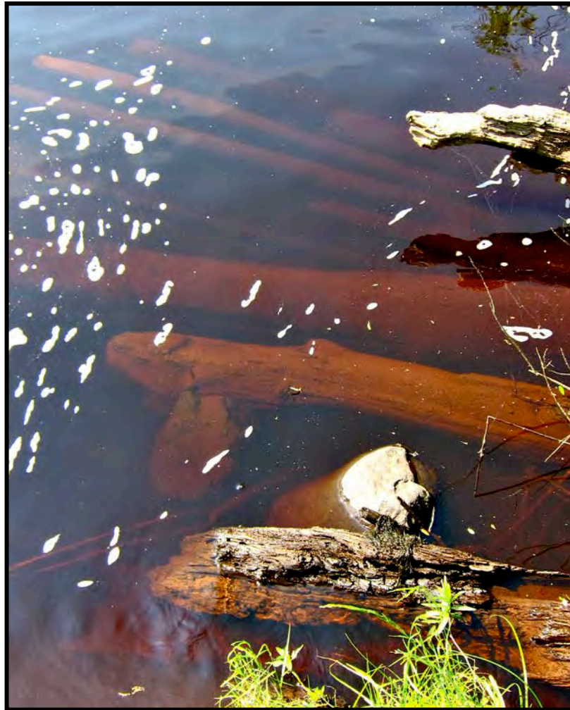
Figure 22: Farthest downstream remains of the log apron at the outlet of a log sluice at the Tamarack Logging Dam (21PN096), facing west on southwest side of ruins. (May, 2013)
