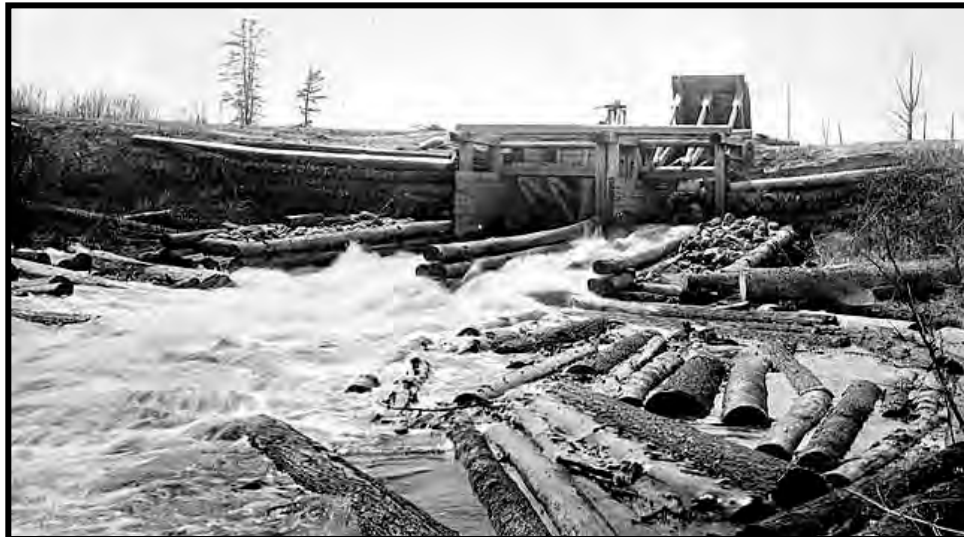
Figure 18: 1912 River Driving Dam at Clam Falls on the Clam River, Wisconsin. The gate on the right is swung up and open. Cribs support the sides of the sluiceways. The dam itself is an earth-filled timber crib that transitions to an earthen dam. The gates are constructed from 8" by 8" timbers. (MHS photo HD5.41 p 22)
