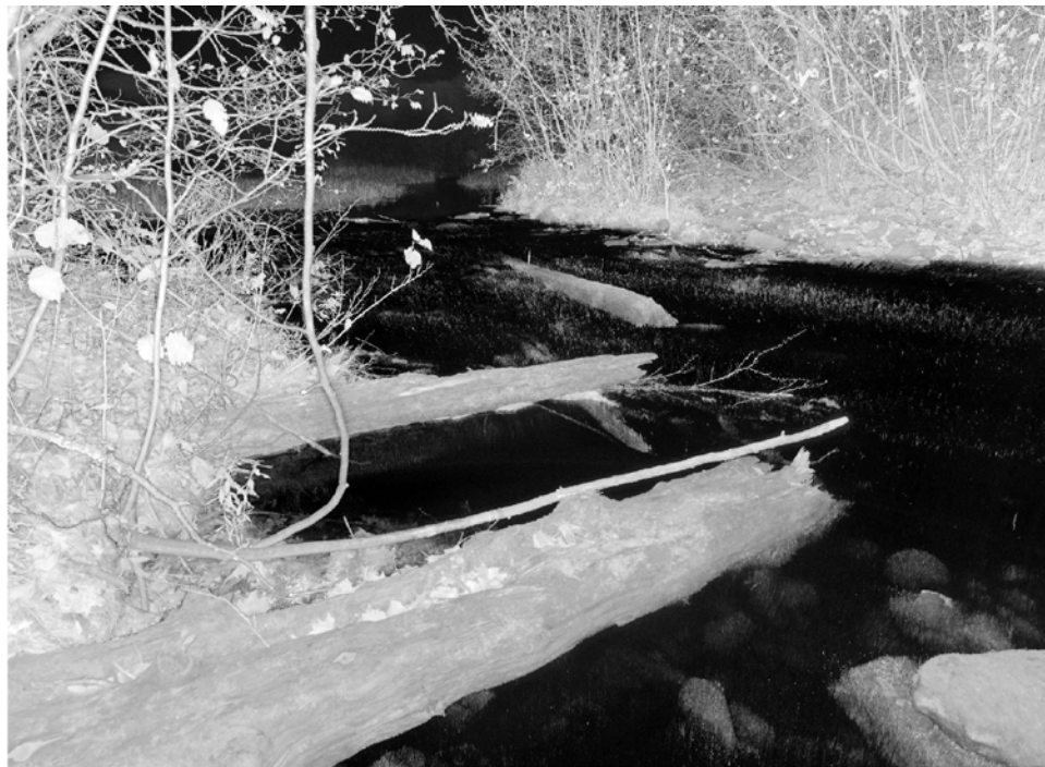
Figure 63. Intensity quick view of the Tamarack Creek Dam (21PN096) sluiceway, looking east.
