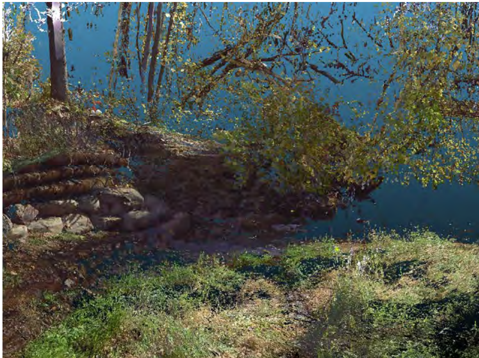
Figure 61. Color 3D view of the Godfrey Dam, looking southeast.
