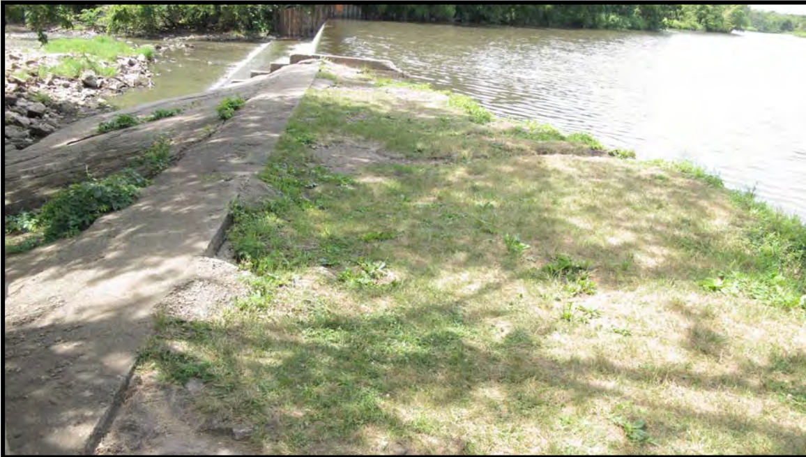
Figure 23: Lake Louise Dam at the former site of the LeRoy Mills facing west. In the foreground the limestone and turf (upstream) and concrete (downstream) facing of the earthen fill dam is visible. The 1925 reconstructed concrete dam is in the background as are the modern sheet piling abutments. August 1, 2013.
