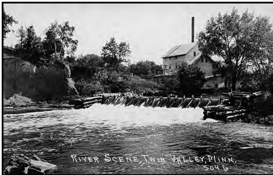
Figure 25: Milldam with timber crib abutments and a plank dam ca 1920. (Minnesota Historical Society Collection negative number 79747)
