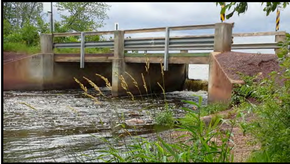
Figure 37: Emily Dam/Bridge in Crow Wing County, Minnesota. Note crest of dam underneath far side of bridge. Construction was sponsored by the state Emergency Conservation Works but funding came from WPA.
