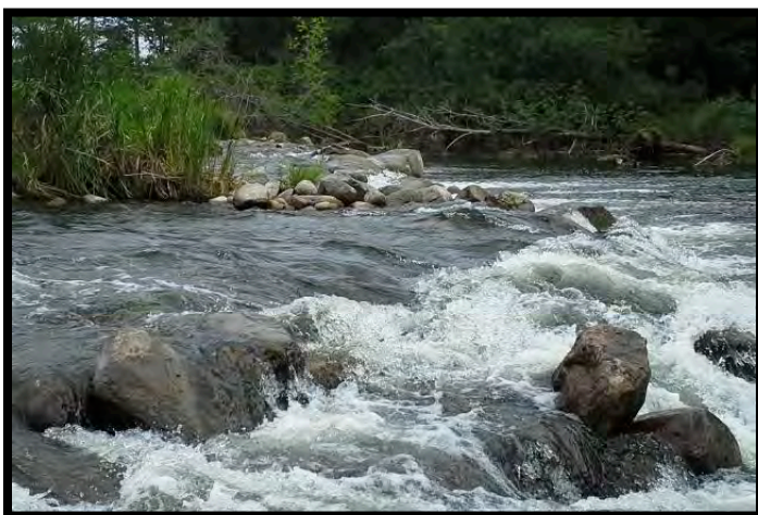
Figure 14: Modern loose rock dam with a head of about 3 feet built to raise lake levels at Pine Lake near Cross Lake, Minnesota for recreation. (July 2013)
