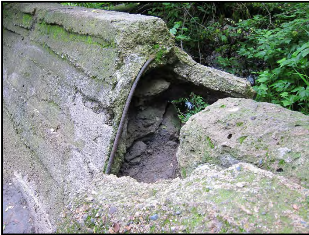
Figure 28: Dam ruins at Zumbrota showing two stages of masonry construction (June 2013)
