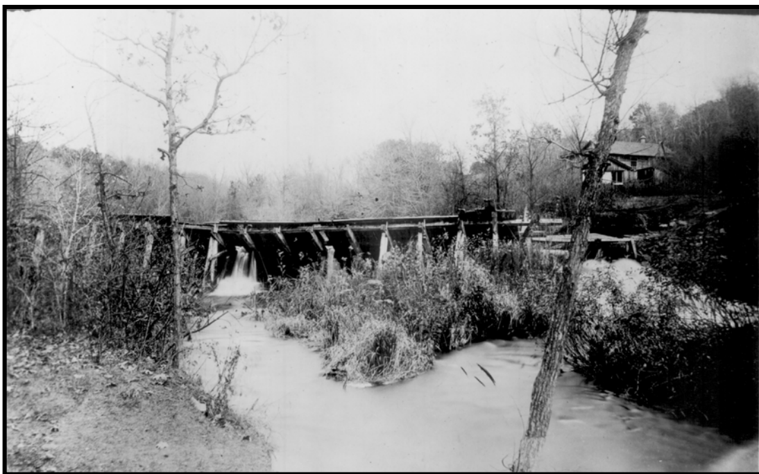
Figure 29: In this photograph of the Godfrey Mill Dam from the 1890s, the plank addition built by Franklin Steele on top of the original masonry dam was falling into ruin. The original limestone base and embankments are still visible at the site.
