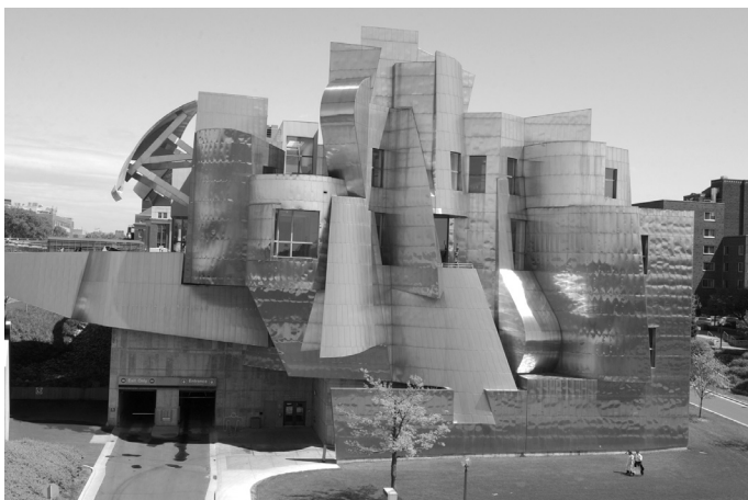
The Weisman Art Museum was designed by Frank Gehry and completed in 1993.
