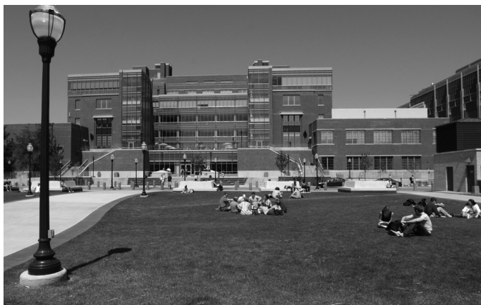
Coffman Memorial Union viewed from the rear, showing the top of the grand staircase that gives access to East River Parkway and the Mississippi River.
