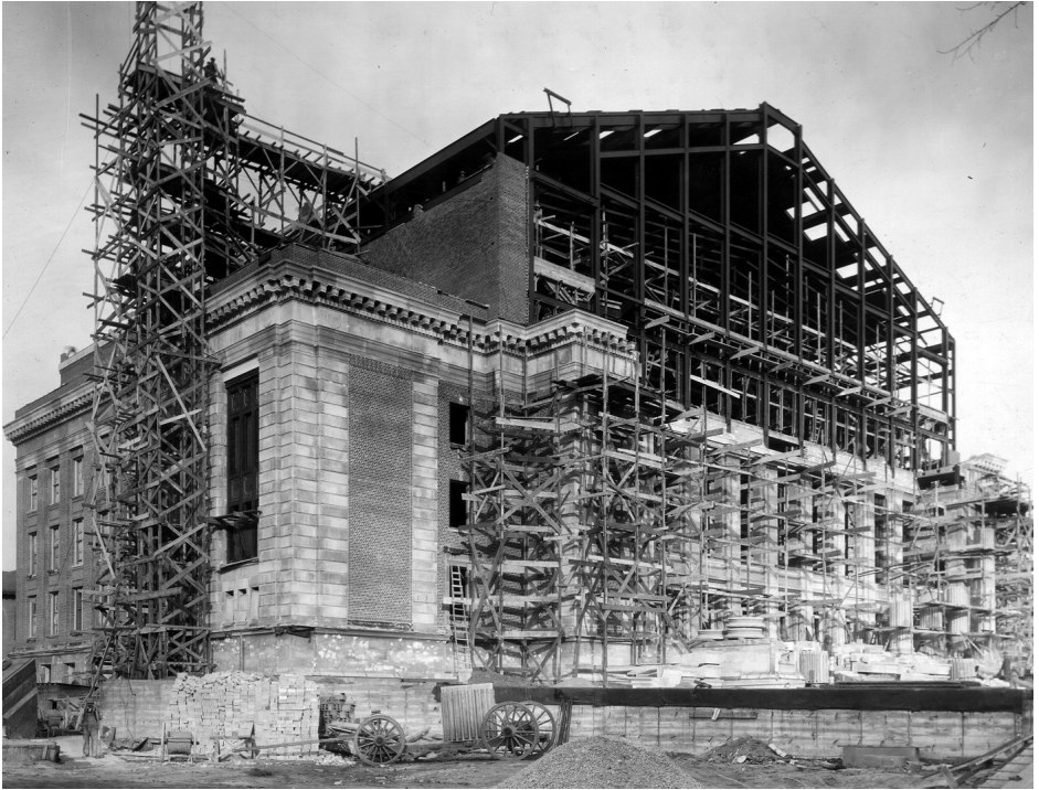
Northrop Hall under construction.
