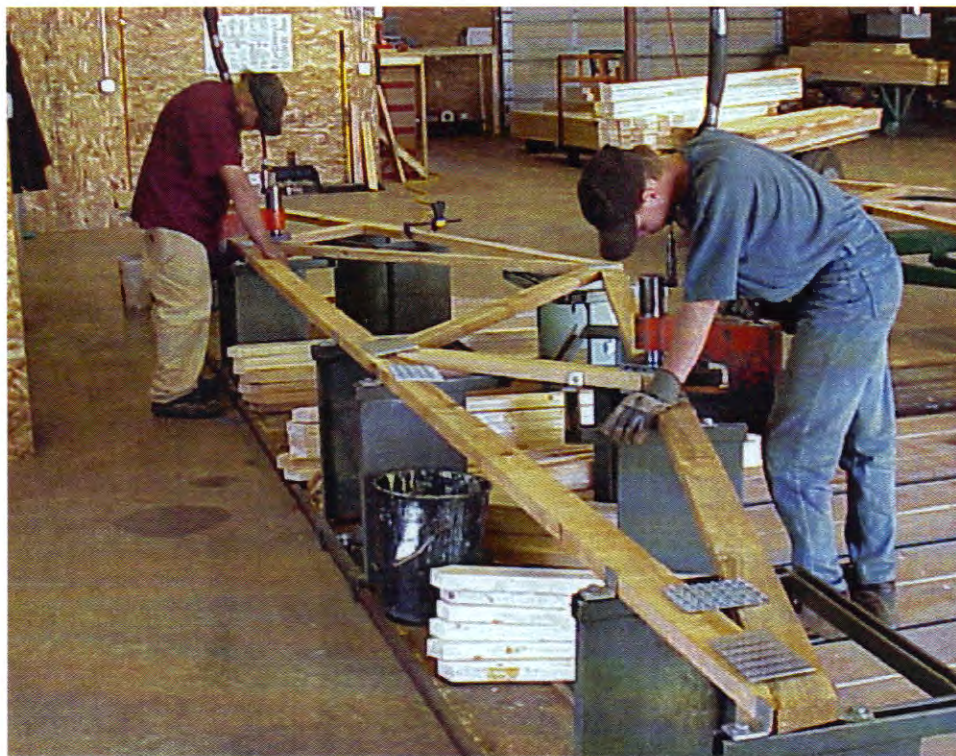
Figure 4.--Hardwood truss manufactured using hydraulic presses.
