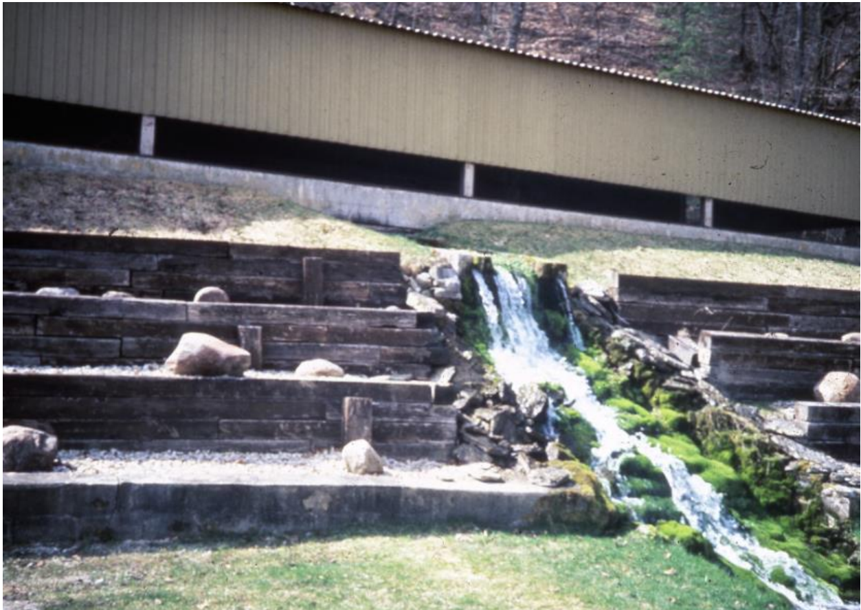
Photo of the Lanesboro Fish Hatchery Main Spring (overflow) (Photo by E. Calvin Alexander, Jr.)
