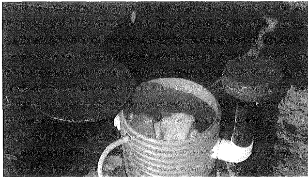
Figure 2. Reactex™ textile filter system installed at NERCC in 1999.
