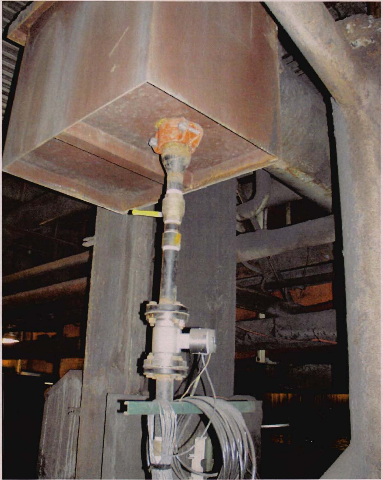
Figure 6 – Close up of Feed Sample Point and Flow Meter
