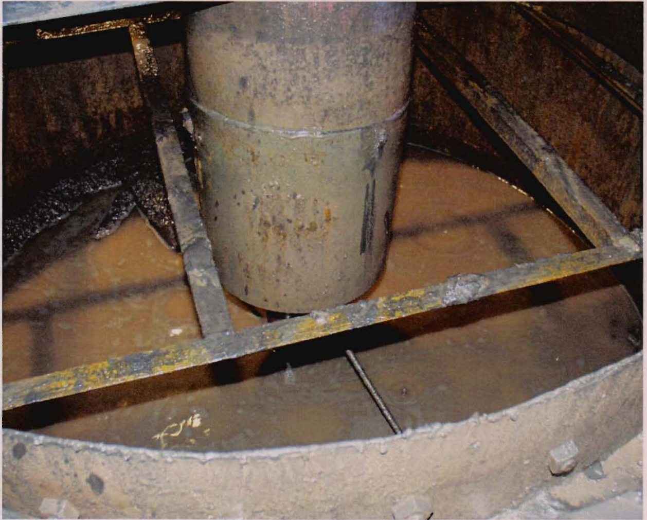
Figure 1 – Steel Supports for Magnet Assembly
