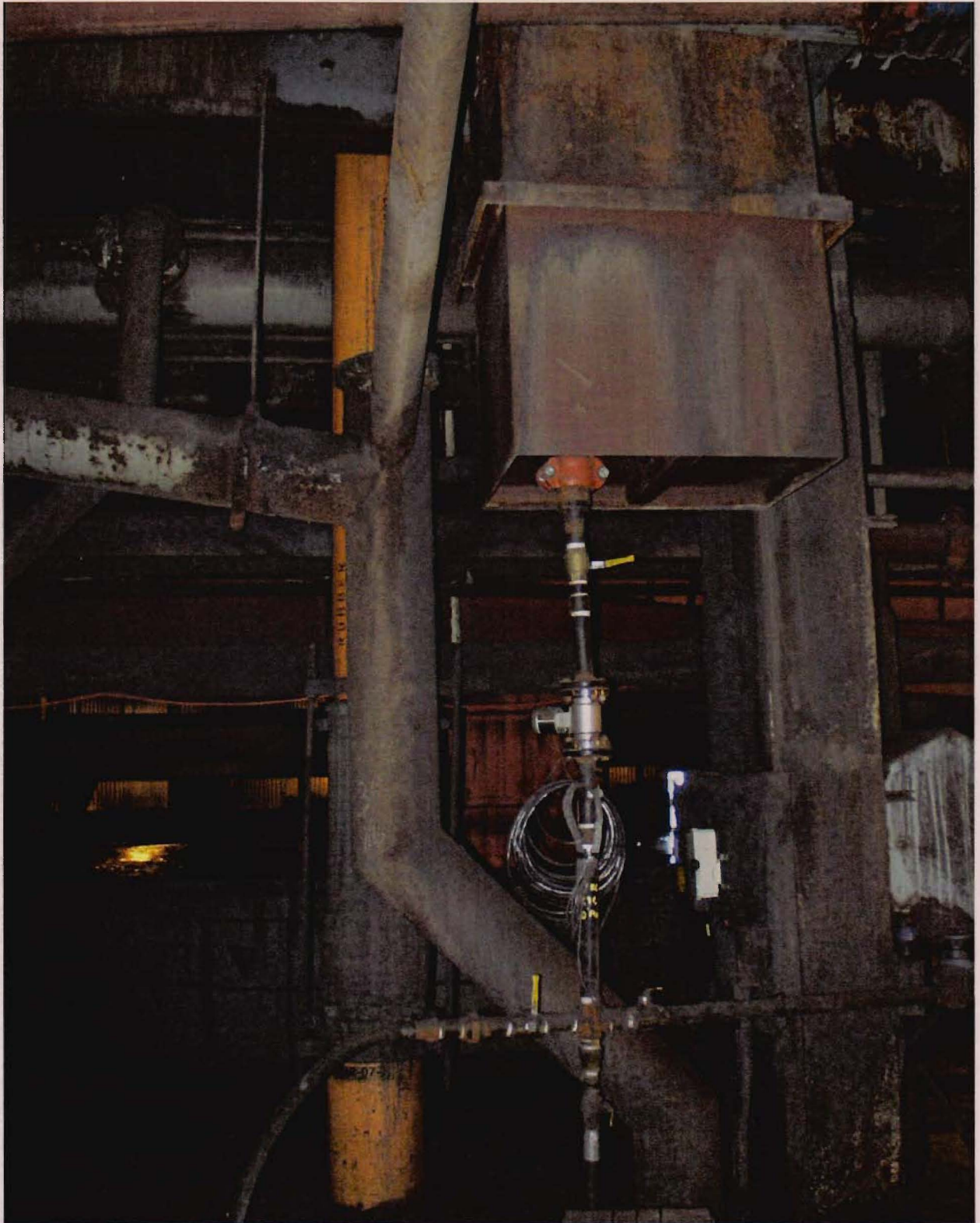
Figure 5 – Feed Line Showing Plant Sample Point and Wash Water Piping
