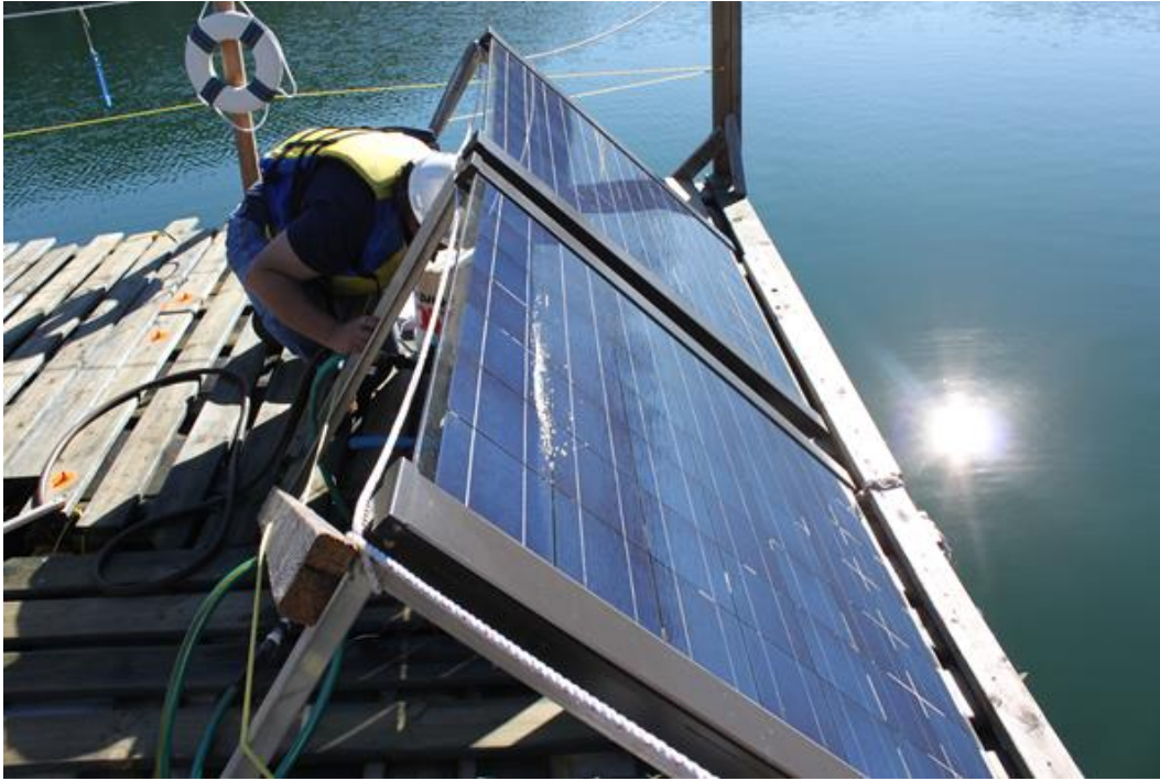
Figure 6. Silicon Energy SiE195 Cascade PV solar panels mounted on the bioreactor raft.
