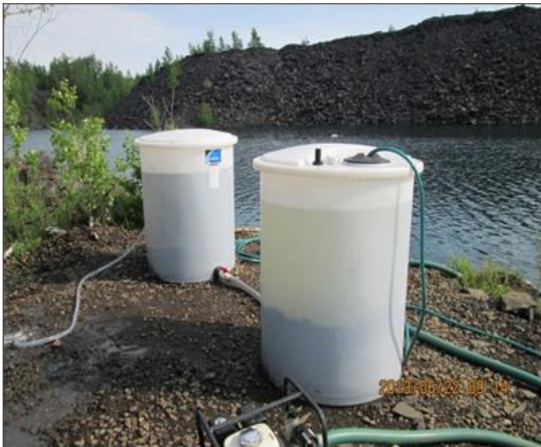
Figure 12. Precipitation tanks initially located on the shoreline in Phase I.
