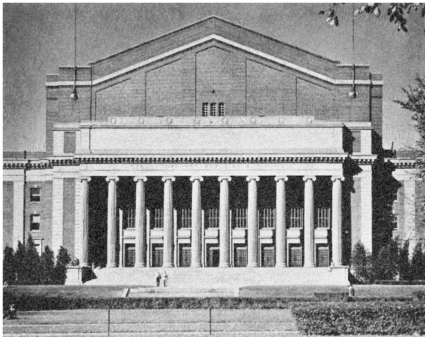
Figure 13 | Northrop Memorial Auditorium front facade. (Source: Photo Files, Northrop Memorial Auditorium Images, University of Minnesota Archives, University of Minnesota, Minneapolis.)
