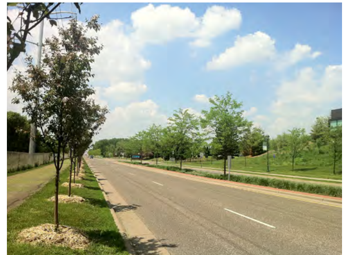
Vegetated median helping calm traffic and providing a pedestrian refuge in Roseville, MN. Photo taken by capstone students.
