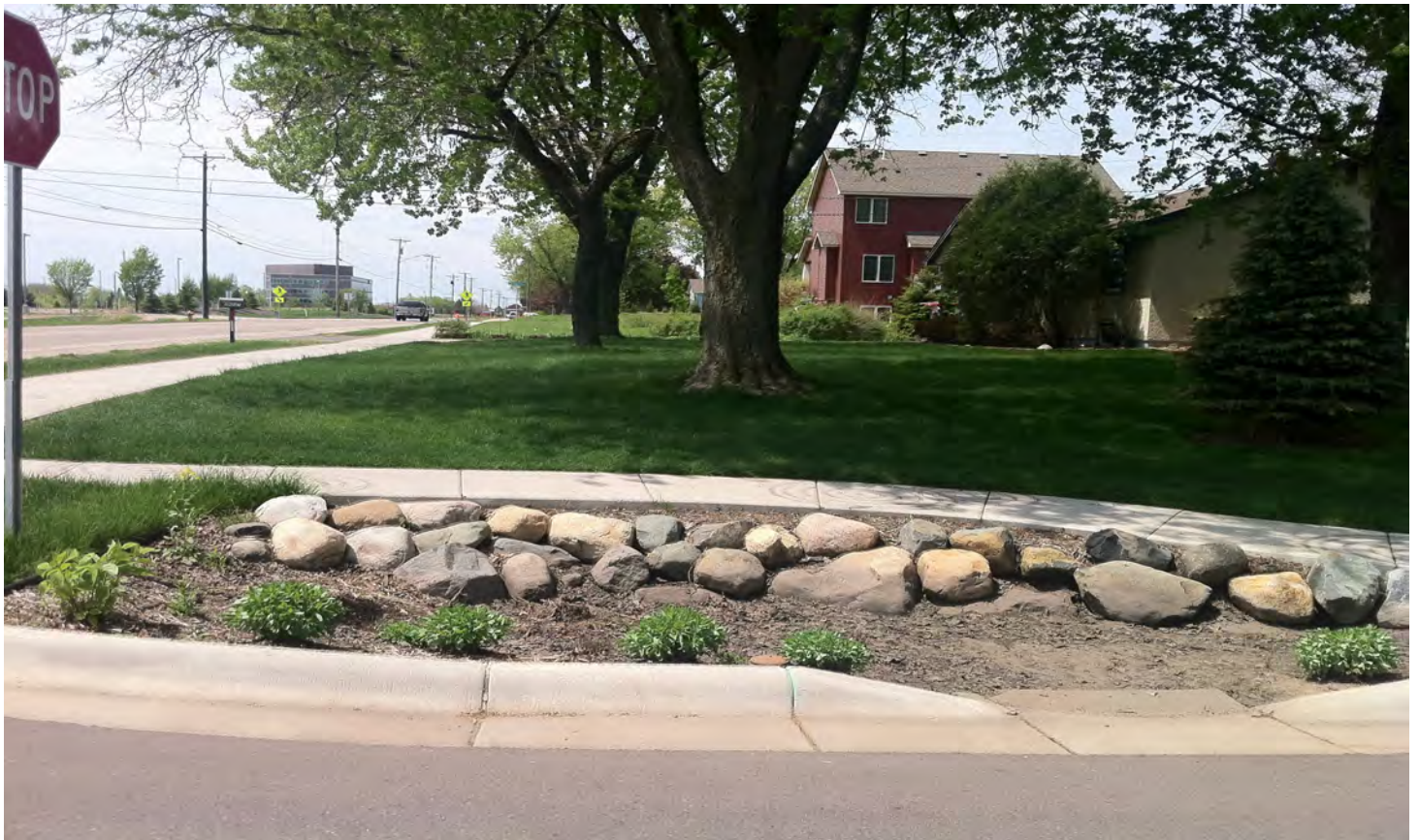
This picture shows a living street in Maplewood, MN. The rain gardens are newly constructed and the plantings are still sparse. Photo taken by capstone students in Maplewood, MN.
