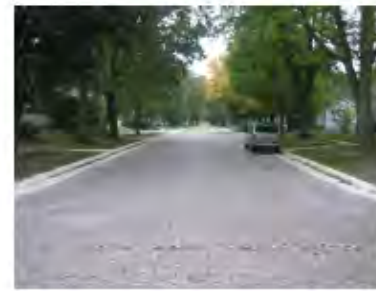
After Permeable Pavement
