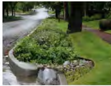
After Raingarden Swale
