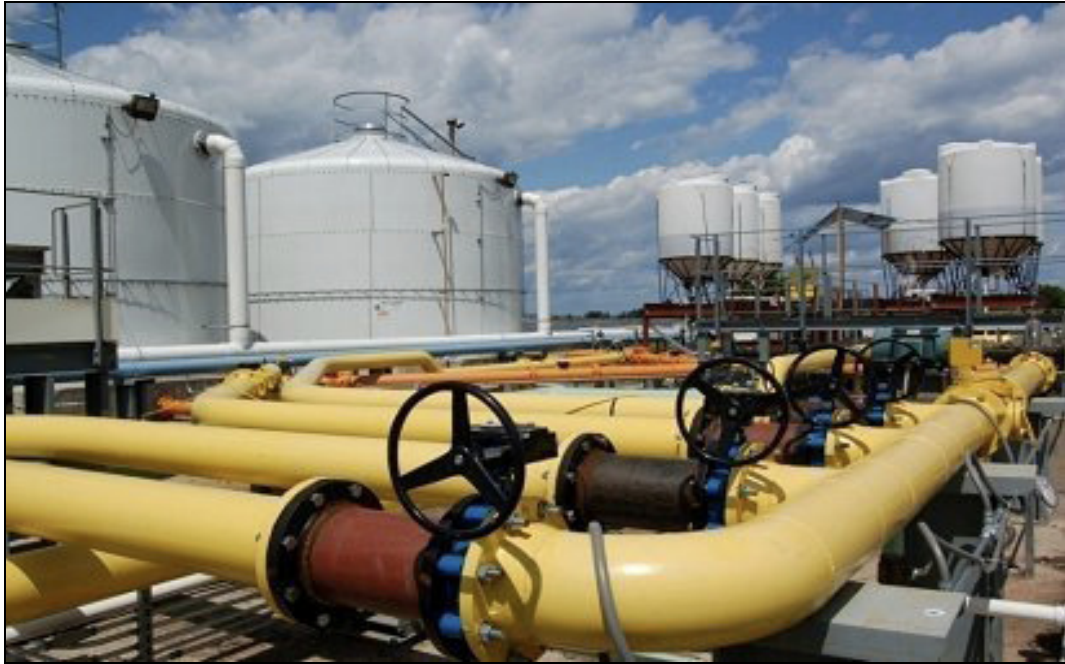
Figure 1. The GSI's Land-Based RDTE Facility in Superior, Wisconsin.
