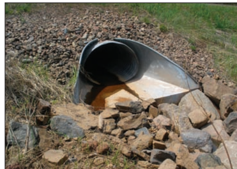
Figure 9: Most efficient, apron outlet
