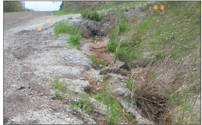
Figure 3: Unstable ditch
