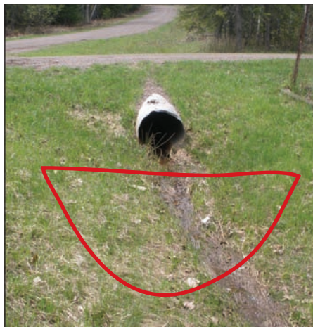
Figure 35: Example of a stable ditch shape
