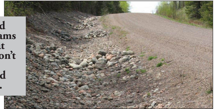
Figure 20: Rock check dam
