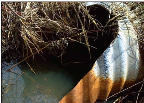
Figure 7: More efficient, mitered cut
