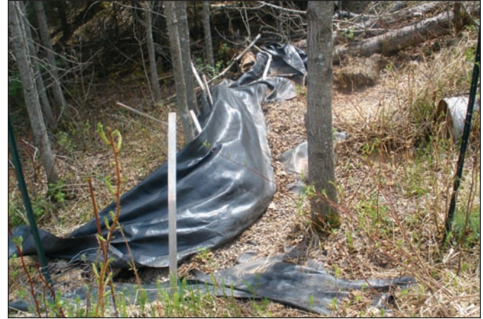
Figure 25: Remove silt fence when vegetation is established
