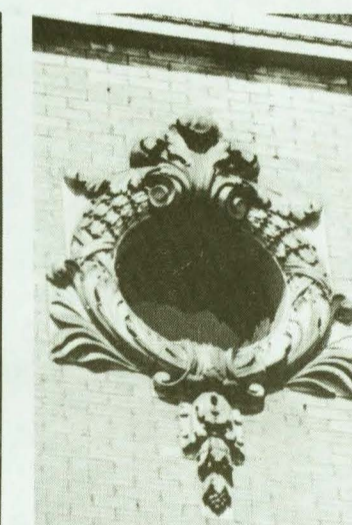
Above: This window on the east side of Old Main is just one of the many architectural details that make the building unique.
