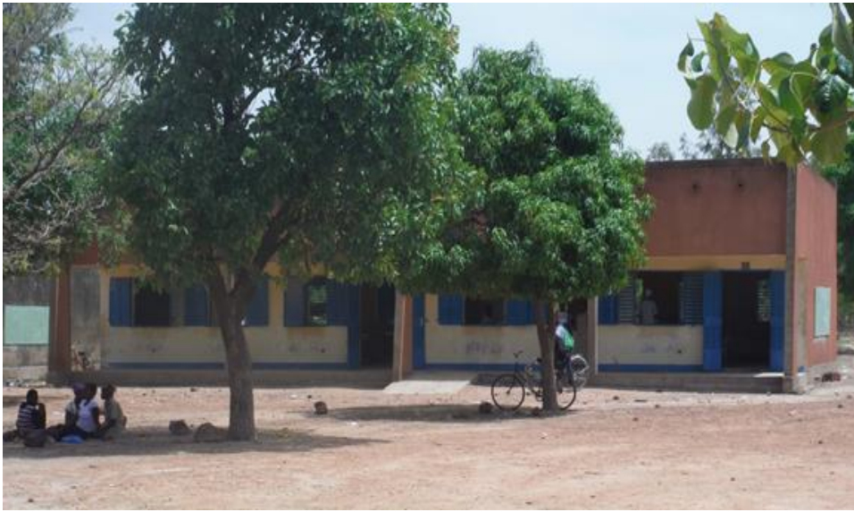
Figure 9. Exterior of classrooms at the Departmental High School of Cassou
