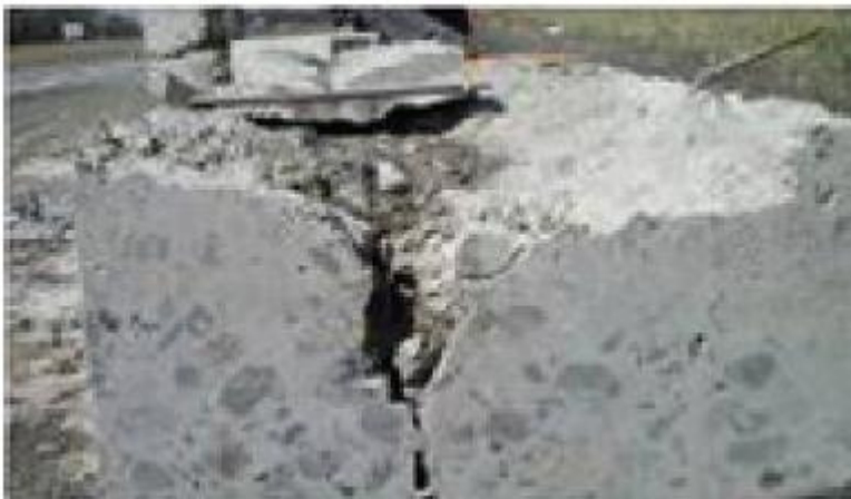
Figure 13: Damaged Joint Detected by MIRA (Hoegh, Khazanovich, and Yu, 2012)
