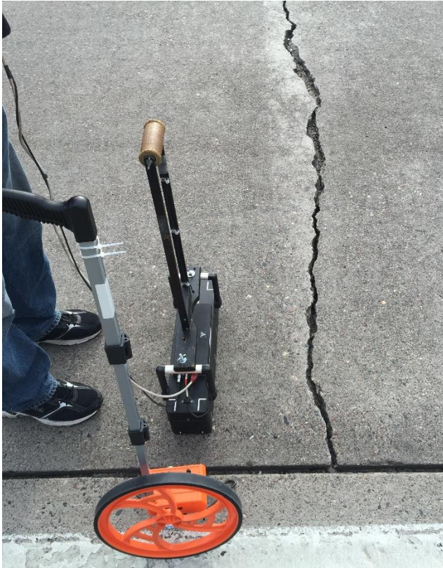
Figure 28: Cracking seen on HWY 60
