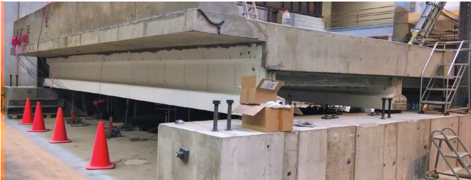
A full-scale single-span bridge with four prestressed concrete girders was constructed in the lab and tested to investigate shear distribution.
