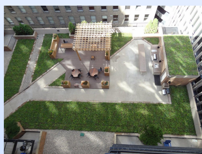
Metro Building Roof, LLC Minneapolis
