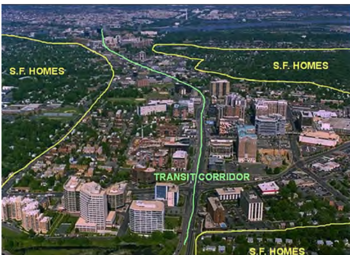
Figure 54. Single family homes are set back from the transit corridor, which is surrounded by higher intensity land uses. Source: http://www.flickr.com/photos/mapei/2601432153/ .
