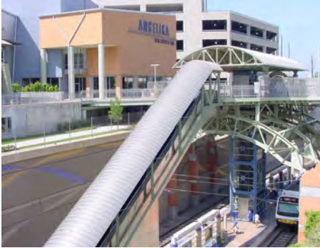
Figure 15. Mockingbird Station's pedestrian bridge provides access to the Mockingbird Station village. Source: http://www.nctcog.org/trans/sustdev/bikeped/access_to_rail/Photos_large/Mockingbird%20Station.jpg .
