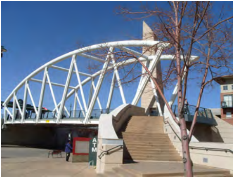
Figure 35. The light rail platforms are adjacent to the BNSF mainline, but the bridge over a series of bus lanes creates a distinctive feature in the plaza area. Source: Author.
