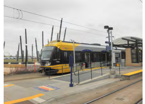
Figure 58. The light rail station interfaces easily with the focal point of Central Park. Source: Author photo.
