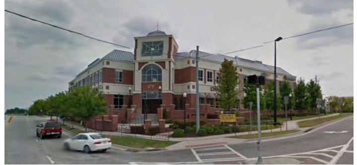
Figure 26. Primary outparcel building, separated from street by berms. Source: Google.
