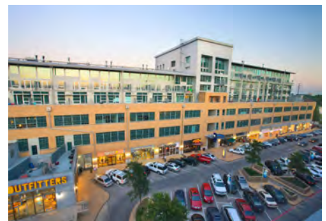
Figure 14. The former Western Electric Building, renovated with additional floors and a brand new roof. Source: http://www.mockingbirdstation.com/info/loftgallery .
