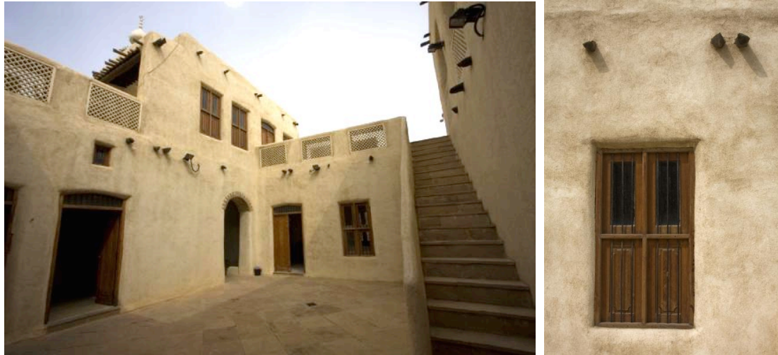
Figure 18. The courtyard of Beit Khalid & wooden window shutters and beams, Kuwait Kester (2016).
