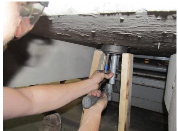
Fig. 3-71 Tapping wedges into the wedge plate
