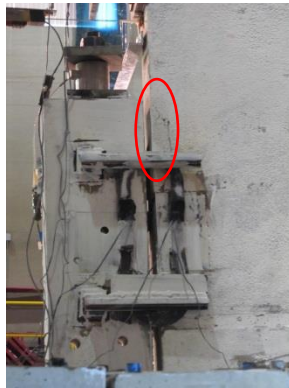
Fig. 7-23 Cracks initiated near the 2 nd story northeast O-connector at 3% drift in Phase 6 (view from north)
