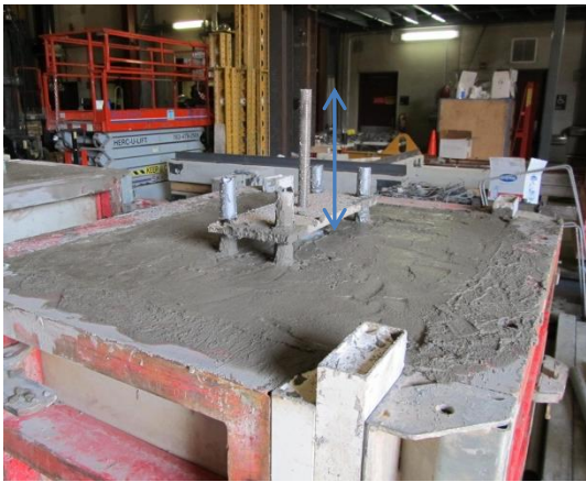
Fig. 3-125 Casting base block of edge columns
