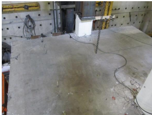
Fig. 6-83 Overall condition of the top surface of the floor slab after the test
