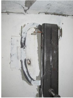
Fig. 6-58 Fractured O-connector at the upper level following the end of the test
