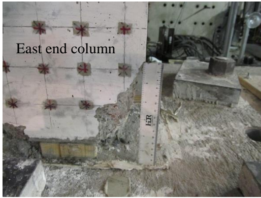
Fig. 7-67 Condition of fiber grout layer beneath the east end column after the test
