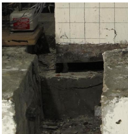
Fig. 6-16 Condition of the fiber grout beneath the west wall corner at 2% drift in Phase 1
