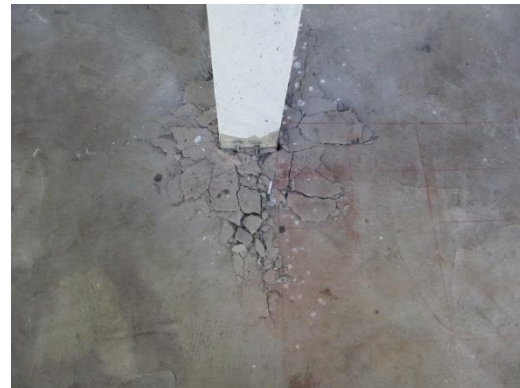
Fig. 6-84 Localized damage at the wall-floor connection after the test
