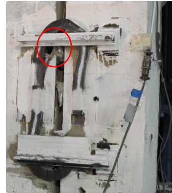
Fig. 7-24 Concrete spalling near the 2 nd story northeast O-connector at 3% drift in Phase 6 (view from south)
