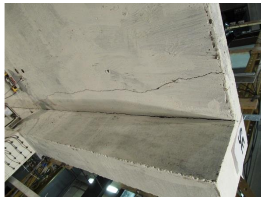
Fig. 6-72 Widely opened cracks at the east floor-edge beam connection in the slab at 2.5% drift in Phase 1 (view from underside of floor)
