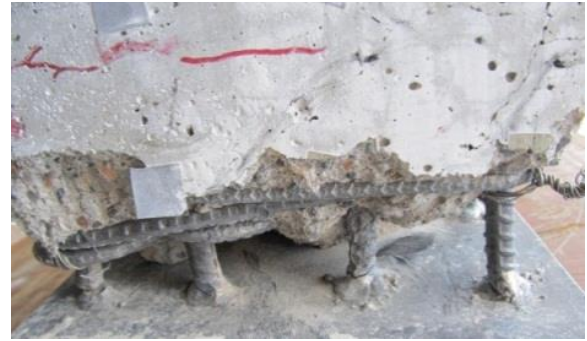
Fig. 7-130 Fracture of the weld for the rebar at the west column base
