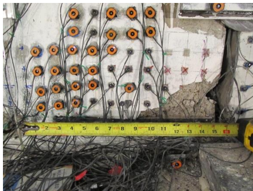
Fig. 7-25 Damage in the east corner of the wall after 5% drift in Phase 7
