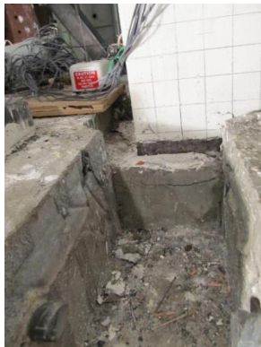
Fig. 8-15 Condition of the west wall corner in PFS1 at 2% drift in Phase 1
