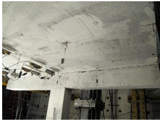
Fig. 6-78 Condition of the bottom surface of the slab after the test
