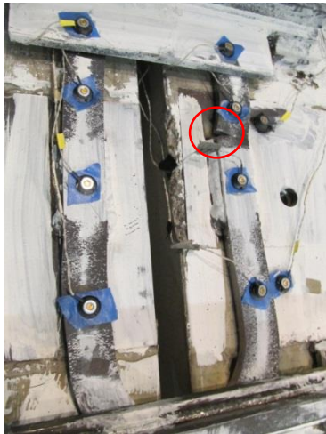
Fig. 7-93 Crack formed near the weld at 4% drift in Phase 5
