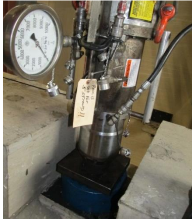
Fig. 3-72 Placement of the post-tensioning jack
