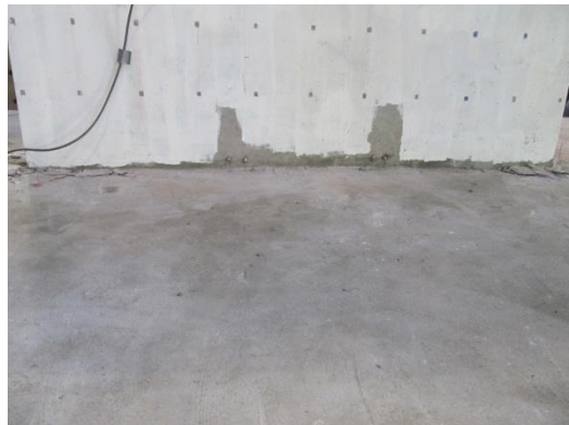
Fig. 6-80 Condition of the top surface of the slab after the test
