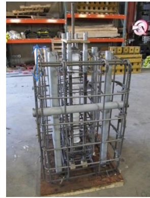
Fig. 3-124 Rebar cage of the base block for edge columns
