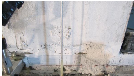
Fig. 7-118 Opening between the base plate and the fiber grout layer at 0.75% drift in Phase 1
