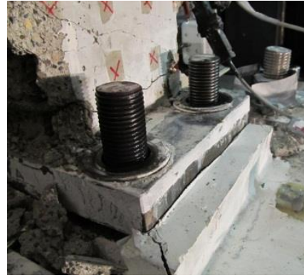
Fig. 7-128 Uplift of the column in Phase 10
