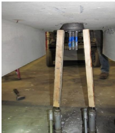
Fig. 3-70 Supporting the bottom wedge plate
