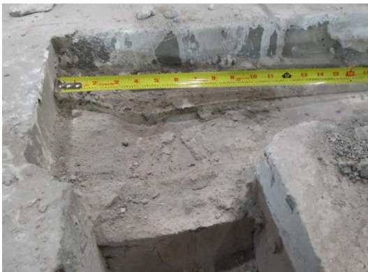
Fig. 8-20 Condition of fiber grout beneath the west corner of the wall after the test of PFS1
