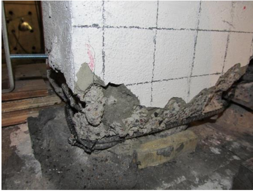
Fig. 7-61 The condition of the west end column after the test (view from south)
