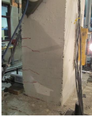
Fig. 6-126 Flexural cracks at the base of the east edge column at 0.25% drift (view from north)
