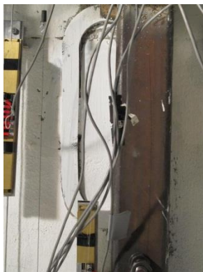
Fig. 6-56 Yield lines on the upper level O-connector at 0.75% drift
