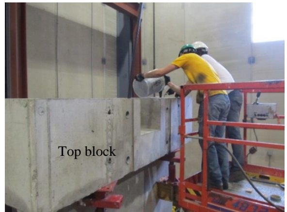
Fig. 3-69 Grouting the rebar in the top block
