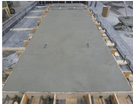
Fig. 3-132 Cast wall in PFS2
