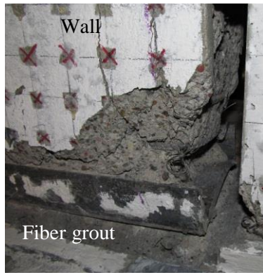
Fig. 7-29 Condition of fiber grout beneath the east corner of the wall after the test
