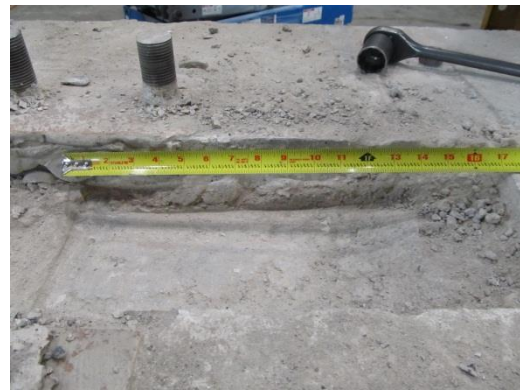
Fig. 8-21 Condition of fiber grout beneath the east corner of the wall after the test of PFS1
