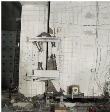
Fig. 7-20 Damage to the concrete cover in the west wall corner at 4% in Phase 5
