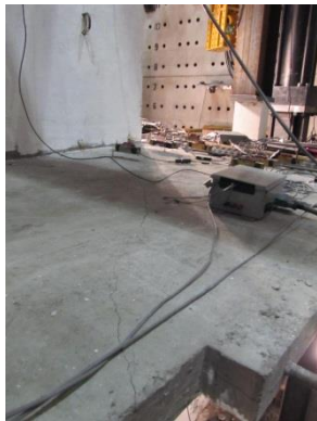
Fig. 6-79 Condition of the damaged top surface of the slab in Phase 3
