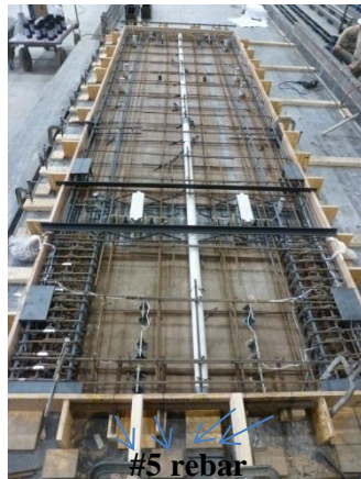
Fig. 3-131 Finished cage for PFS2 wall
