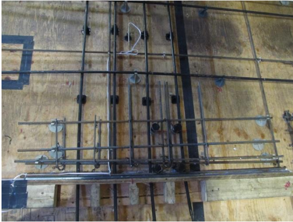
Fig. 3-29 Anchorage zone of the transverse strands
