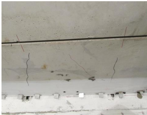
Fig. 7-103 Cracks in the south middle plank at 0.75% drift in Phase 3
