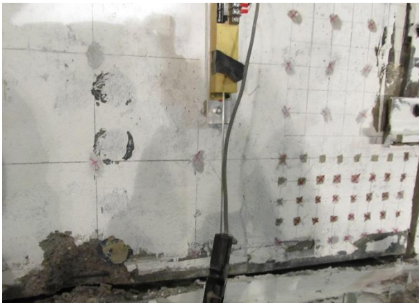
Fig. 7-18 Concrete over spalling in the wall at -2% drift in Phase 2
