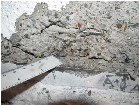
Fig. 7-123 Fracture of the weld of the rebar observed at 4% drift in Phase 5
