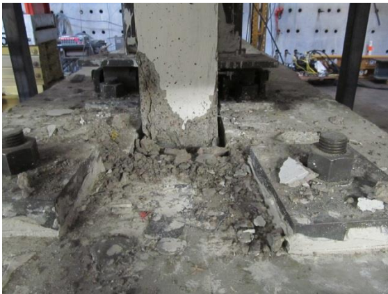
Fig. 6-19 Condition of the east wall corner after the test
