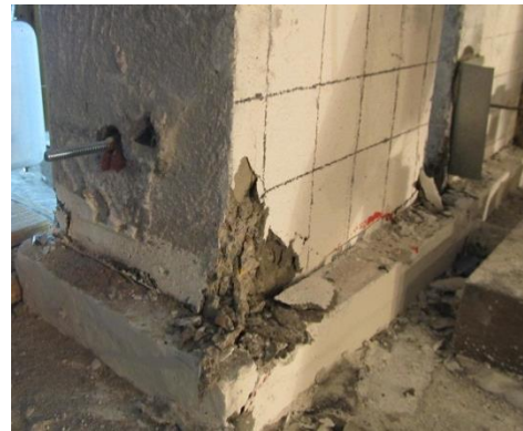
Fig. 7-64 Damage of the fiber grout beneath the west corner of the west end column at -2% in Phase 2 (view from south)
