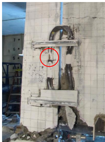
Fig. 7-95 "Half-fractured" O-connector at 5% drift in Phase 8
