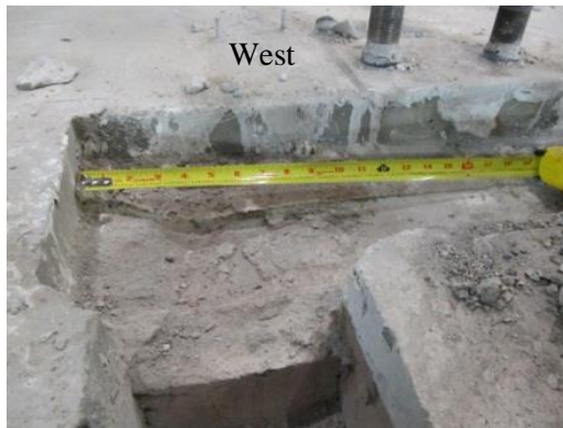
Fig. 6-31 Condition of the fiber grout layer beneath the west and the east wall corner
