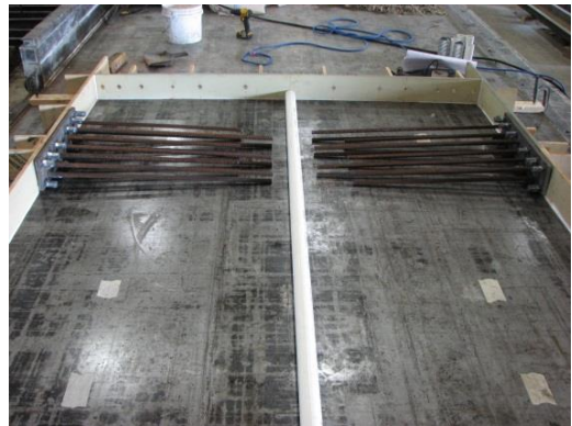
Fig. 3-60 Steel embedment at top of the wall
