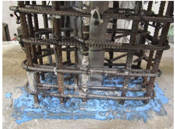
Fig. 3-56 Weldcrete at the base of the column
