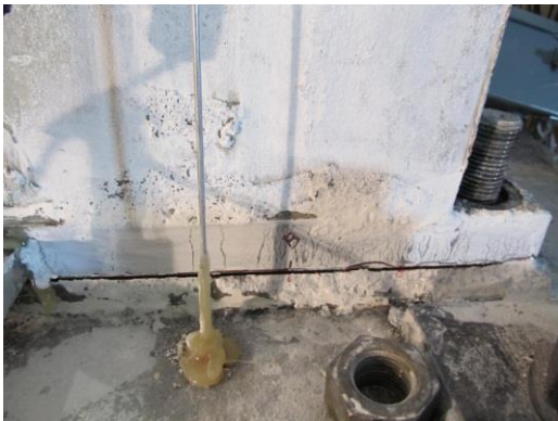
Fig. 7-119 Opening between the base plate and the fiber grout at 2% drift in Phase 1
