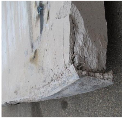
Fig. 9-4 Bending of the steel angle in the wall at the end of the test of PFS1
