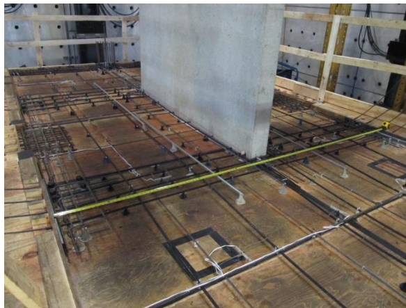
Fig. 3-33 Layout of the reinforcement and strands of the floor slab before casting
