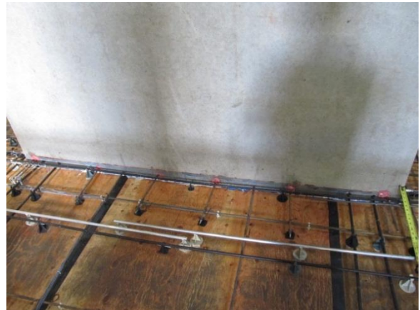
Fig. 3-75 Temporary aluminum rods for leveling the surface of the slab
