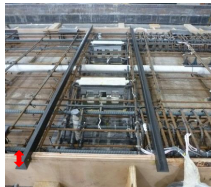
Fig. 3-128 Extended side formwork of wall
