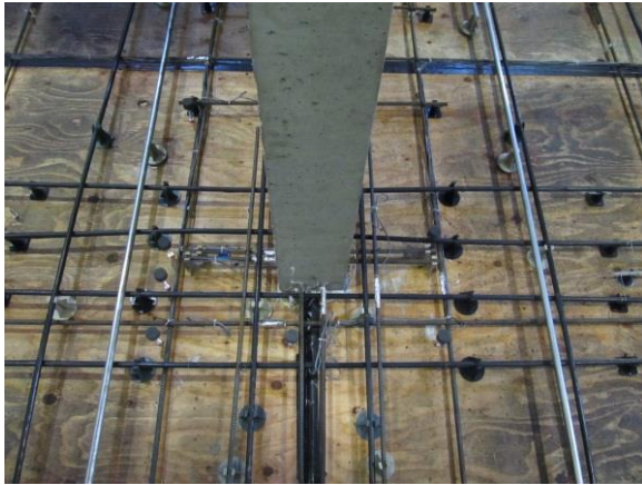
Fig. 3-31 Strand and rebar layout at the wall-floor connection
