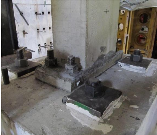
Fig. 3-141 Finished edge column base
