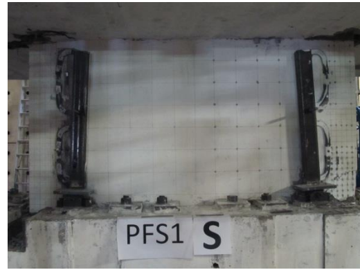
Fig. 8-18 Condition of the wall panel after the test of PFS1
