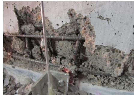
Fig. 7-126 Conditions of the east edge column after 5% drift in Phase 8
