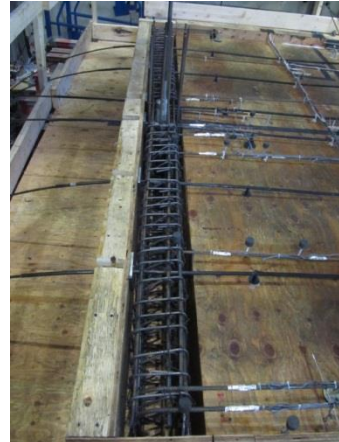
Fig. 3-30 Bonded rebar at floor-column connection
