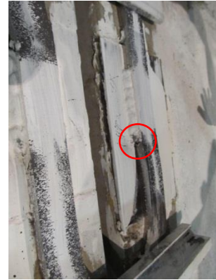
Fig. 7-92 Crack initiated at the weld of the O-connector
