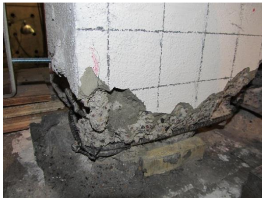
Fig. 8-26 Condition of the fiber grout beneath the west end column after the test of PFS2
