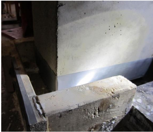
Fig. 3-137 Formwork for grout
