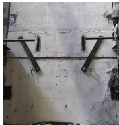
Fig. 3-134 Slotted channel before the test
