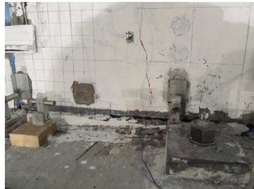
Fig. 8-16 Condition of the west wall corner in PFS2 at 2% drift in Phase 1
