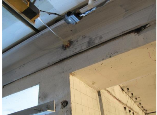
Fig. 7-62 Tensile cracks in the bottom of the transverse beam at 3% drift in Phase 6
