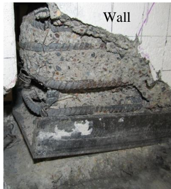
Fig. 8-22 Condition of the fiber grout beneath the west wall corner after the test of PFS2
