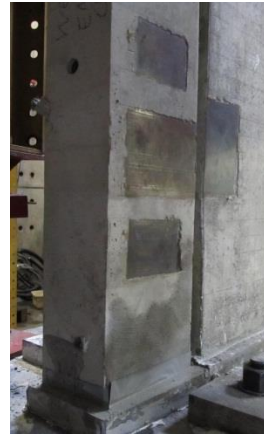
Fig. 3-138 Cured fiber grout layer
