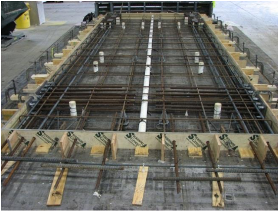
Fig. 3-63 Finished steel cage of the wall
