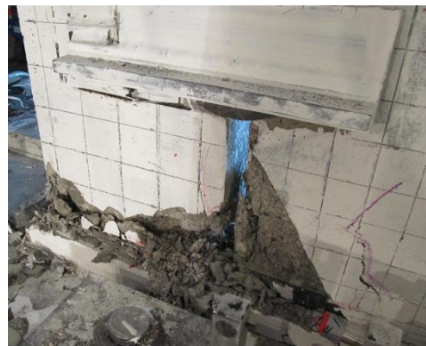
Fig. 7-58 Damage to the west end column at the peak of 5% drift in Phase 7
