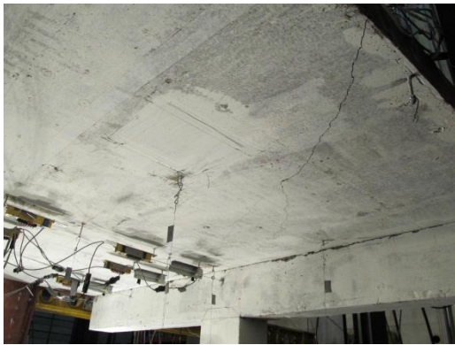
Fig. 6-77 Condition of the damaged bottom surface of the slab in Phase 3
