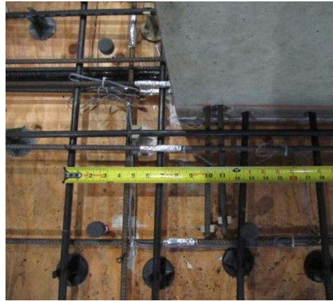
Fig. 3-32 Strand and rebar of the slab running through the wall
