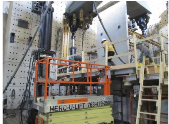
Fig. 3-77 Casting the PT floor slab
