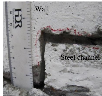
Fig. 7-26 Separation between the steel channel and the concrete in wall corner
