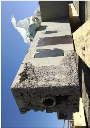
Fig. 3-135 Concrete consolidation
