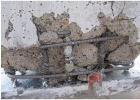
Fig. 7-129 Crushing of the concrete core and fracture of the rebar at the east column base
