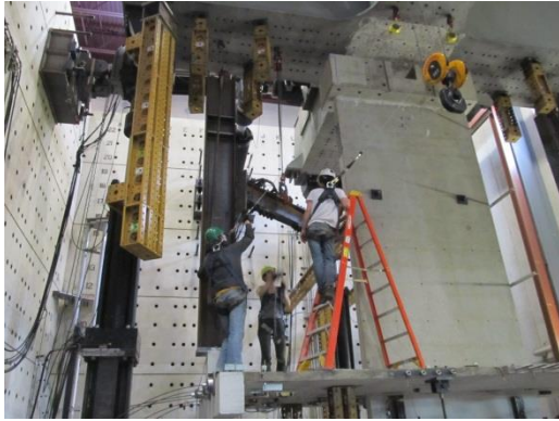
Fig. 3-84 Installing the mega beam
