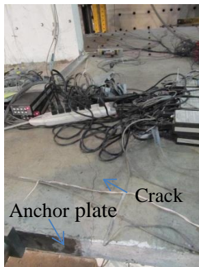
Fig. 6-71 Cracks in the slab extending to the end of the common anchor plate in Phase 1 (view from top of floor)
