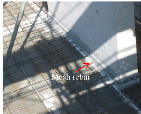
Fig. 2-40 Wall-slab connection in the transverse direction (Nagae et al. 2011)
