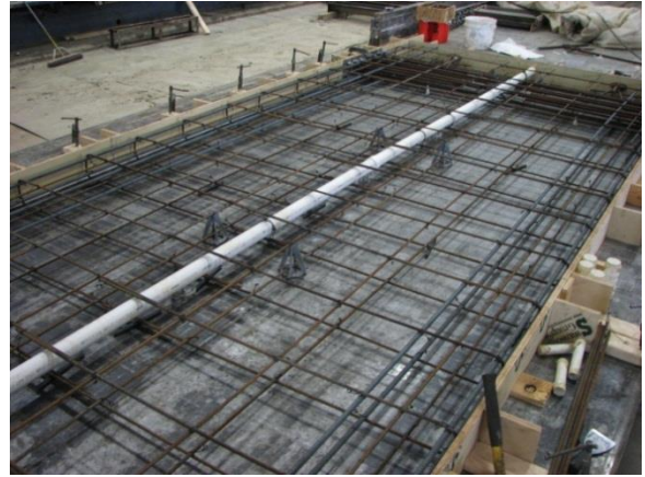
Fig. 3-62 Mesh reinforcement in the wall
