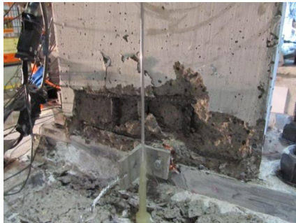
Fig. 7-125 Damage to the east edge column base at 2% butterfly loading in Phase 6
