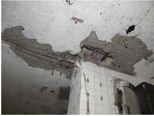
Fig. 6-75 Localized damage at the west wall-floor connection in Phase 3 (view from underside of floor)
