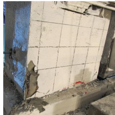
Fig. 7-52 Damage in the west corner of the west end column at -1.5% drift in Phase 1
