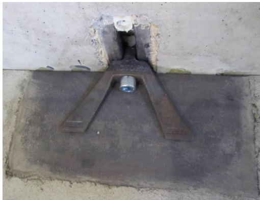
Fig. 3-145 BS Italia before welding
