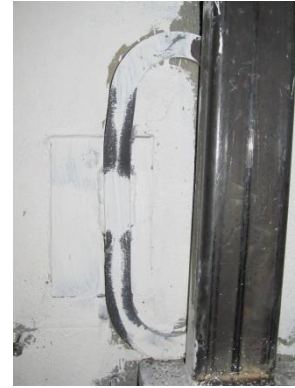
Fig. 6-59 Uncracked O-connector at the lower level following the end of the test
