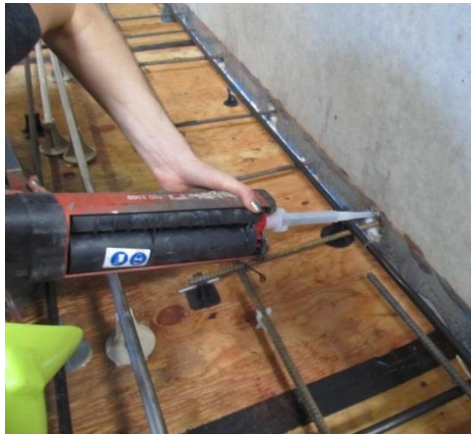
Fig. 3-74 Injecting mortar to grout reinforcement through the wall
