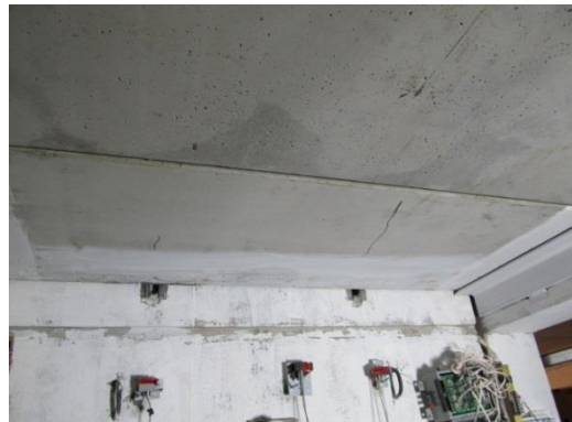
Fig. 7-104 Cracks in the north middle plank at 0.75% drift in Phase 3
