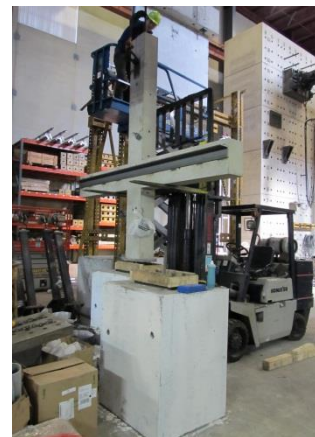
Fig. 3-140 Installation of edge column
