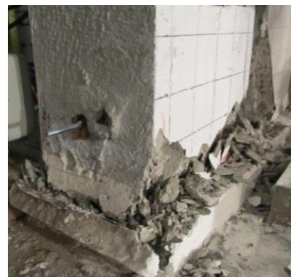
Fig. 7-66 Spalling of the upper corner of the fiber grout beneath the east corner of the east end column at 2.5% in Phase 5
