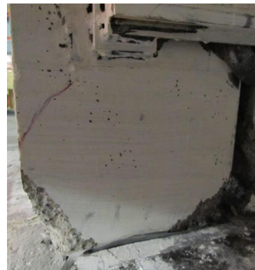
Fig. 7-60 The condition of the east end column after the test (view from north)
