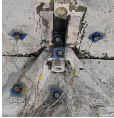
Fig. 7-105 Condition of the BS Italia connection at 4% drift in Phase 5
