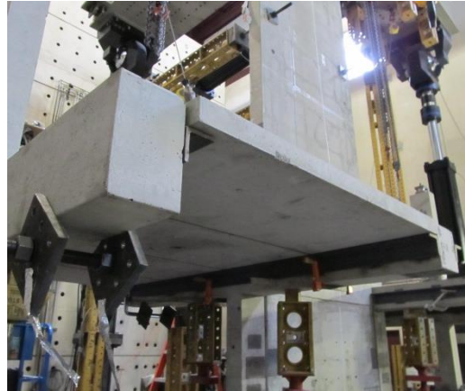
Fig. 3-142 Installation of precast planks
