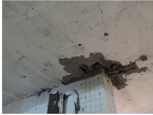
Fig. 6-76 Localized damage at the east wall-floor connection in Phase 3 (view from underside of floor)
