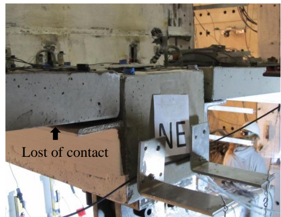
Fig. 7-90 Contact loss between the planks and the steel angle affixed to the transverse beam
