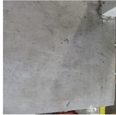
Fig. 6-82 Condition of the slab at floor-edge beam connection after the test
