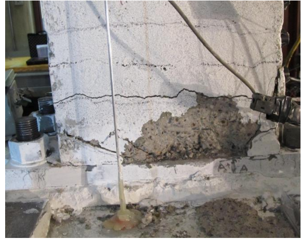
Fig. 7-122 Crushing of the concrete cover in the edge column at 4% drift in Phase 5
