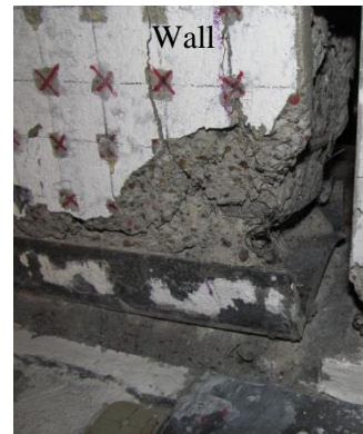
Fig. 8-23 Condition of the fiber grout beneath the east wall corner after the test of PFS2
