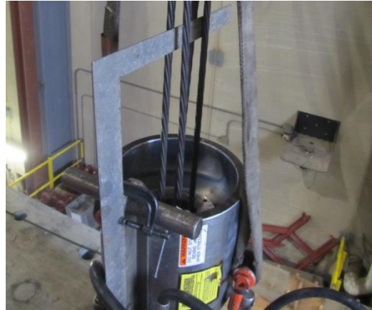
Fig. 3-73 Measuring elongation of the strands
