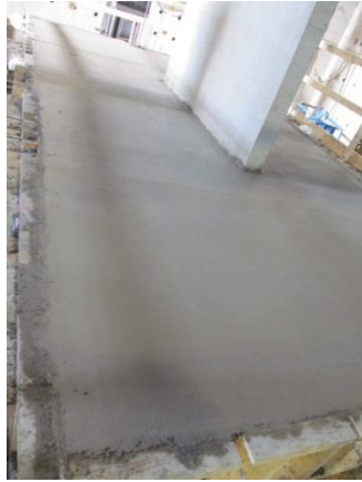
Fig. 3-78 Finished floor slab
