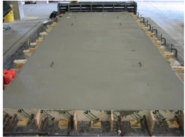
Fig. 3-64 Cast wall panel
