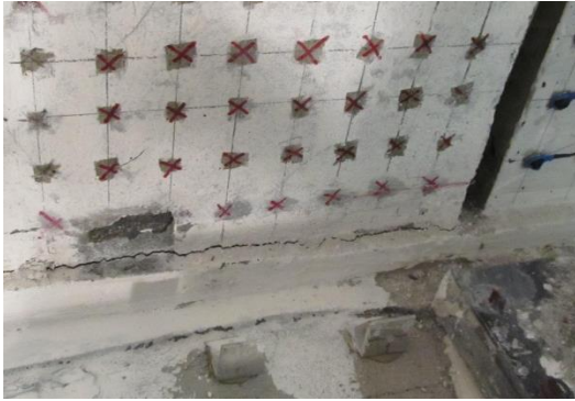
Fig. 7-16 Horizontal crack at the east wall corner at -0.25% drift (view from south)
