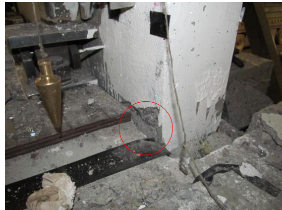
Fig. 6-20 Condition of the west wall corner after the test
