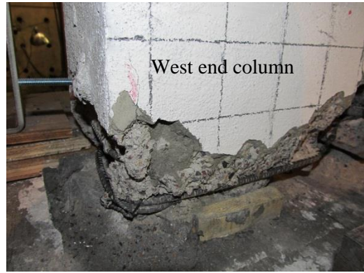
Fig. 7-68 Condition of fiber grout layer beneath the west end column after the test
