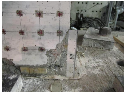
Fig. 8-27 Condition of the fiber grout beneath the east end column after the test of PFS2
