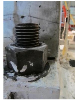
Fig. 7-124 Separation between the edge column and the base plate at 4% drift in Phase 5
