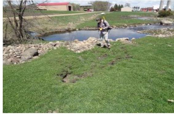
The longest hydrologically connected SPI signature of the top 1% of values in the study area was along Mill Creek (pictured above left). The accompanying field photo shows signs of slumping in the small pasture (foreground) and the landowner had installed rip-rap along the stream bank for stabilization. There was no further evidence of erosion upland of the slumping.
