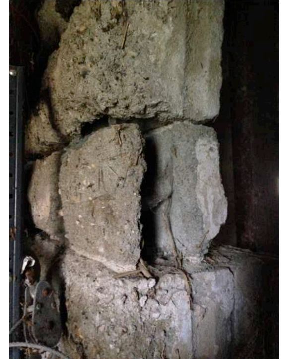
1.11 South silo wall CMU contains course, large aggregate with sandy mortar. Missing mortar in this area
