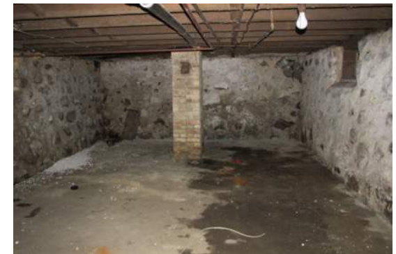
New Basement- View of North Chimney
