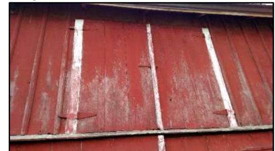
Fig. 6: Upper swing doors. Photo taken facing south.
