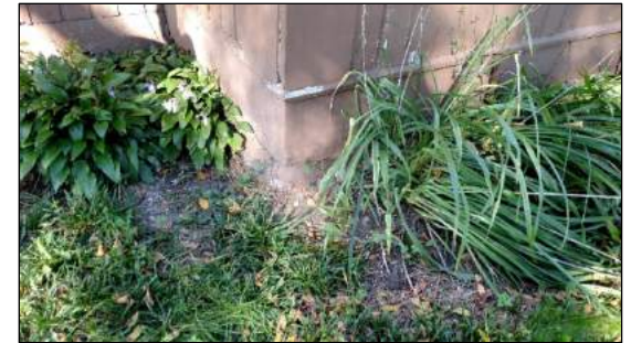
Fig. 6) Detail of foundation and siding baseboard. Photo taken facing northwest.
