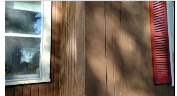
Fig. 2) Detail of the transition from the central main house siding on the right and the southern enclosed porch siding on the left. Photo taken facing west.
