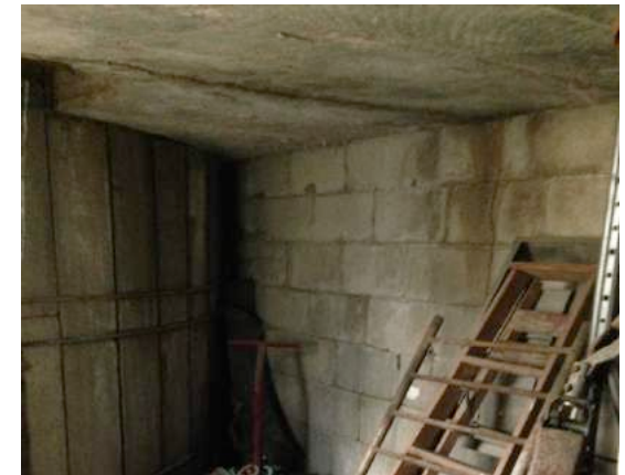
1.11 South silo wall CMU contains course, large aggregate with sandy mortar. Missing mortar in this area
