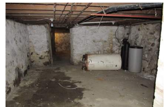
New Basement- View to the South
