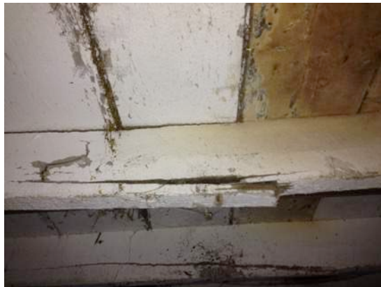
1.9 Joist fracture
