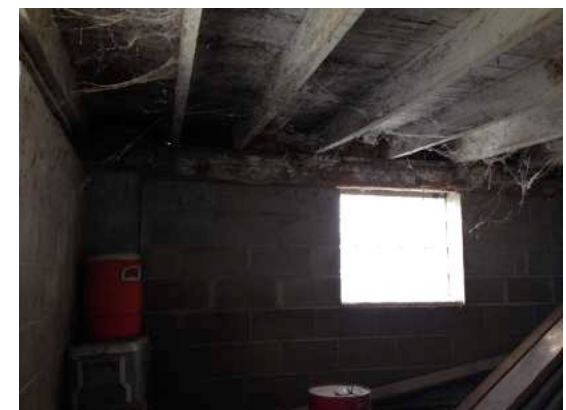
1.10b CMU condition at East Corner
