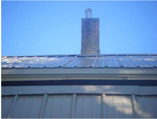
Figure 4: Chimney and roof of farmhouse
