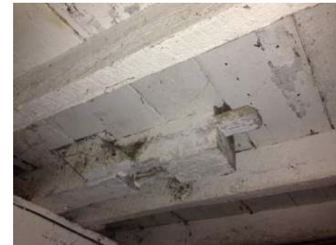
1.23 Bracing Timber attaches to joist in lower level
