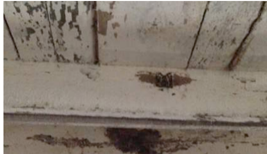
1.4 View of center of joists with metal connection
