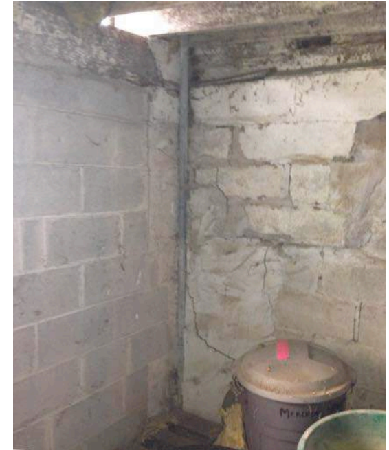
1.10a CMU condition at West corner
