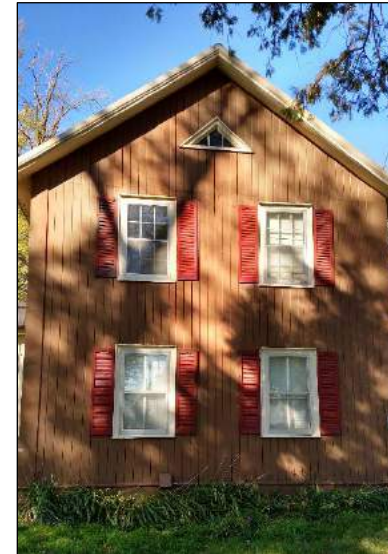
Fig. 4) Central main house section. Photo taken facing west.
