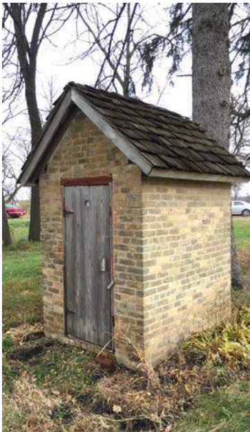
Figure 1: Southwest Elevations of Smokehouse
