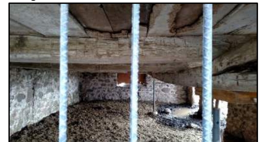
Fig. 12: Interior of lower level. Photo taken facing east.
