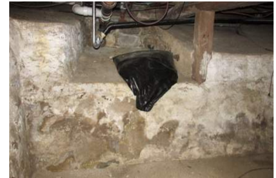
Original Basement- West Wall
