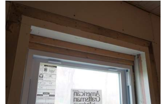
Window 5a- Wood Filler at Head
