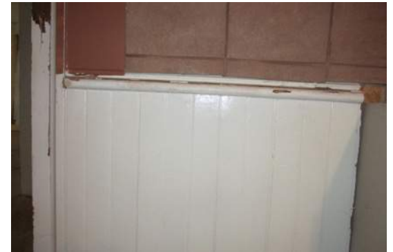
Room 3- South Wall Chair Rail and Door 3-2
