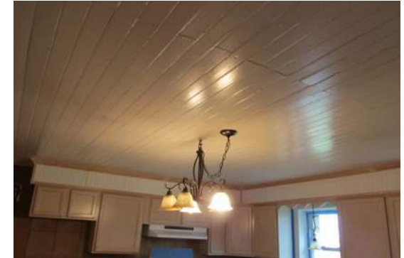
Room 3 Central Ceiling
