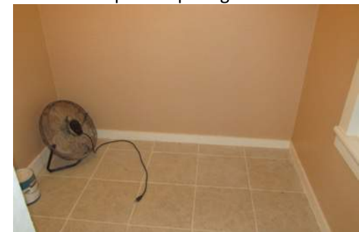
Room 2 Tile and Walls
