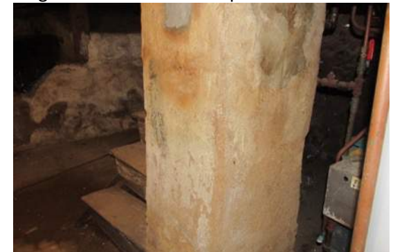
Basement- South Chimney
