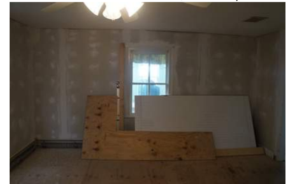
Room 6- South Wall
