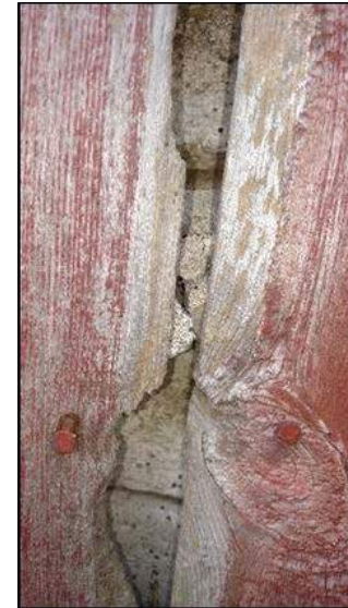
Fig. 7: Exposed inner hand-hewn log structure. Photo taken facing south.
