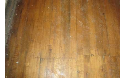
Room 3 Floor, West
