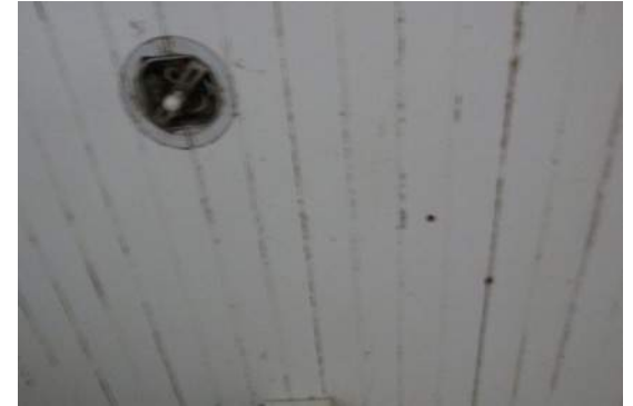
Room 7- Bathroom Ceiling Light
