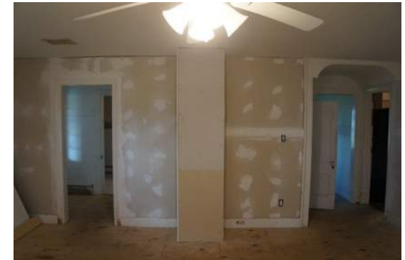
Room 6- View West of Walls, Chimney
