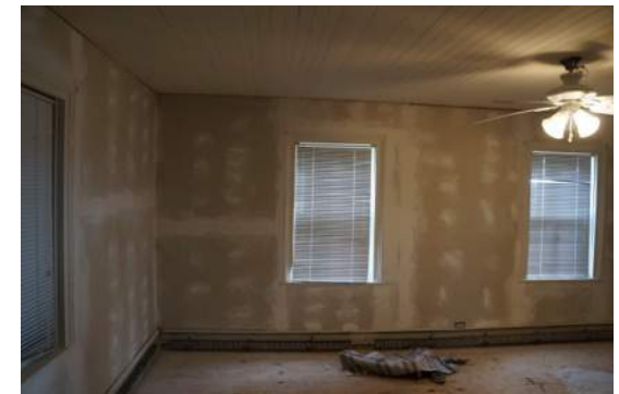
Room 6- East Wall
