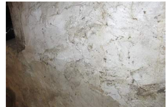
Original Basement- Foundation Wall
