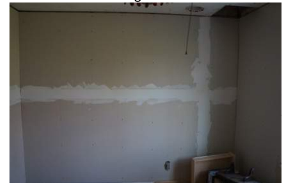
Room 5- South Wall
