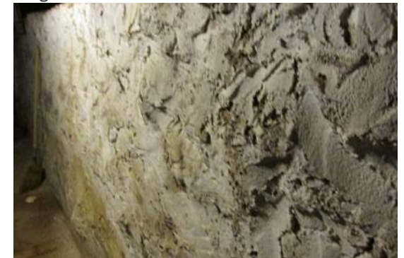
Original Basement- Foundation
