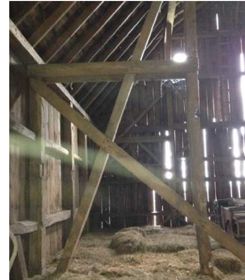
1.22 Loft Bracing Timbers
