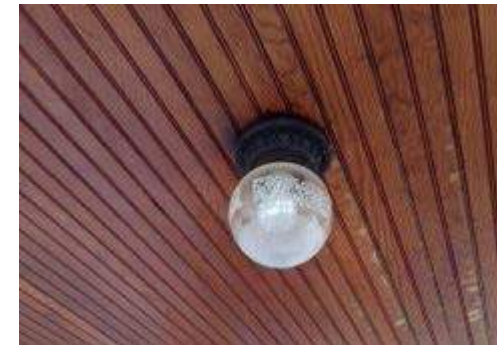
Figure 23. The beadboard ceiling is in good condition.
