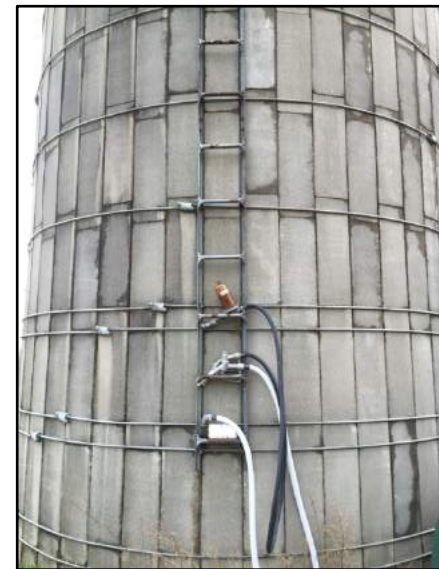
Figure 14: The concrete silo.
