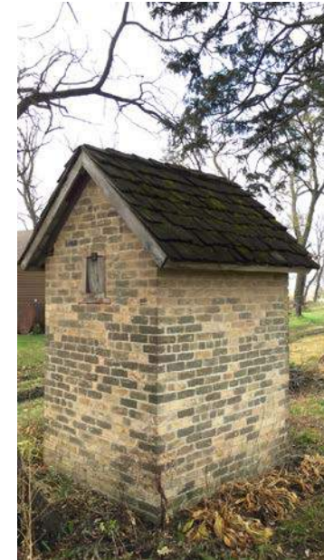
Figure 2: Northeast Elevations of Smokehouse
