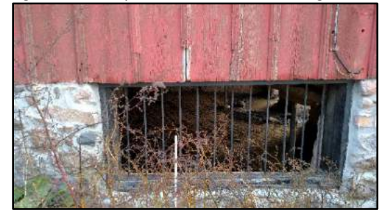
Fig. 11: Foundation window opening. Photo taken facing east.
