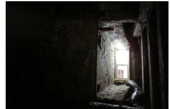
Original Basement- East Window
