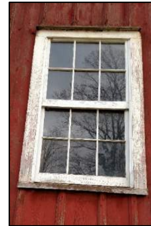
Fig. 10: First story window. Photo taken facing east.
