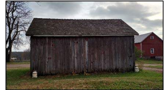
Fig. 2: West façade. Note South Barn in the background.
