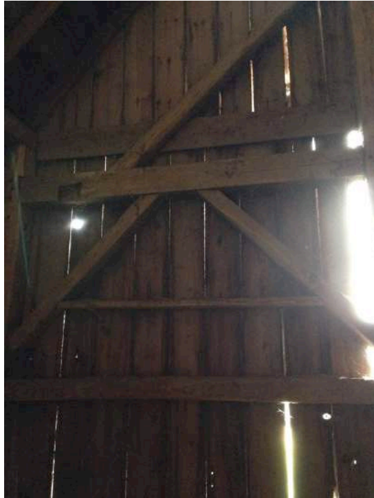
1.17 East Loft Wall
