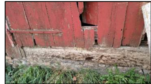
Fig. 8: Hand-hewn beam door sill. Photo taken facing south.
