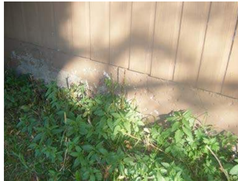
Figure 2. Concrete foundation wall of porch.
