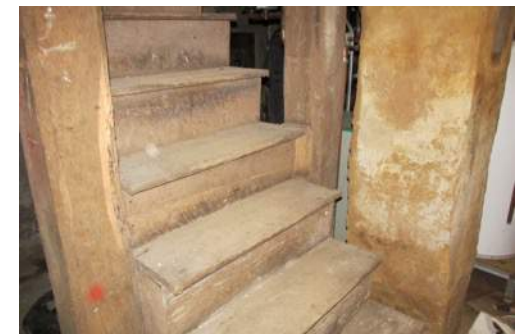
Basement Main Stairway
