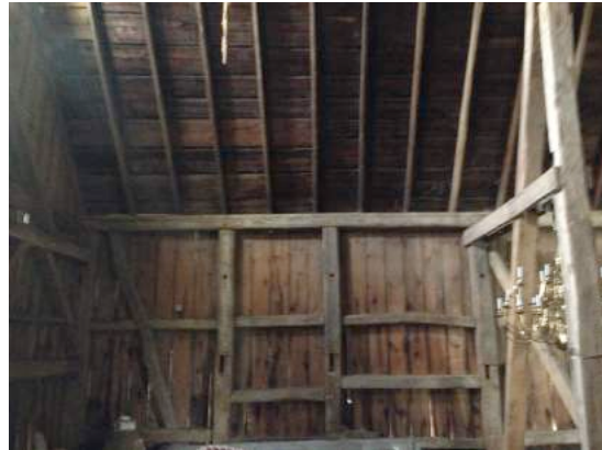
1.20 South Loft Wall
