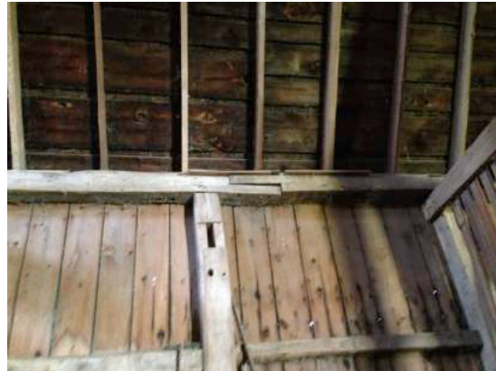
1.21 Loft Wall to Roof Connection
