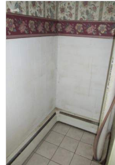
Room 7- Southwest Corner, Wall and Heater
