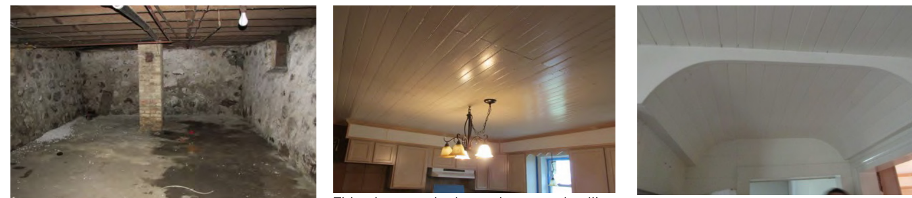
New Basement. view of North Chimney. Photograph shows standing water on the floor. There is rising damp on the first few feet of the basement caused by water infiltration. It is recommended that the ground is regraded along the exterior of the farmhouse in order to decrease the amount of infiltration and prevent further damage.
