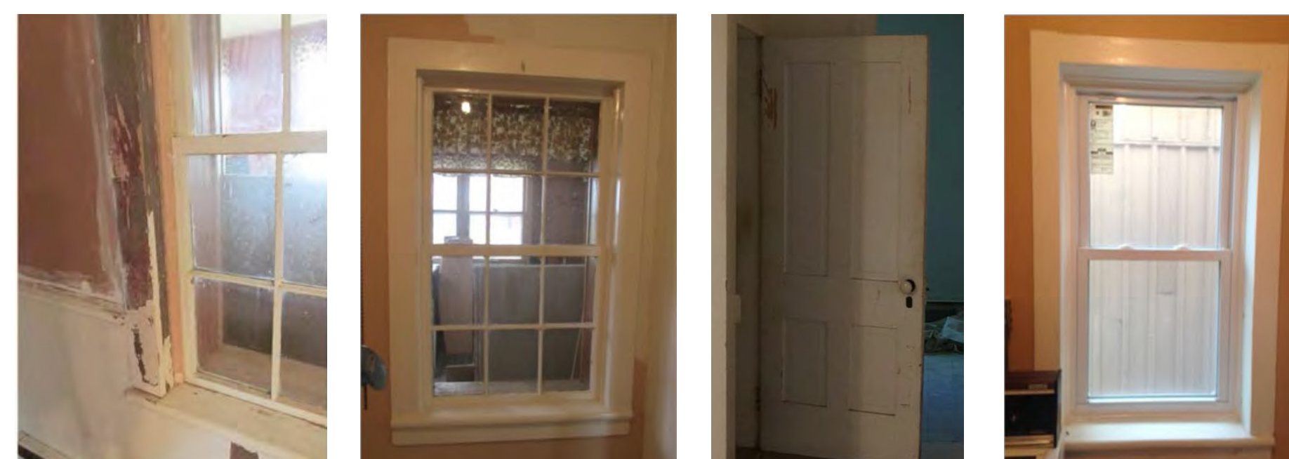
The original trim on this window in the kitchen is in good condition, but should be repainted to a historically appropriate color based on paint sampling.
