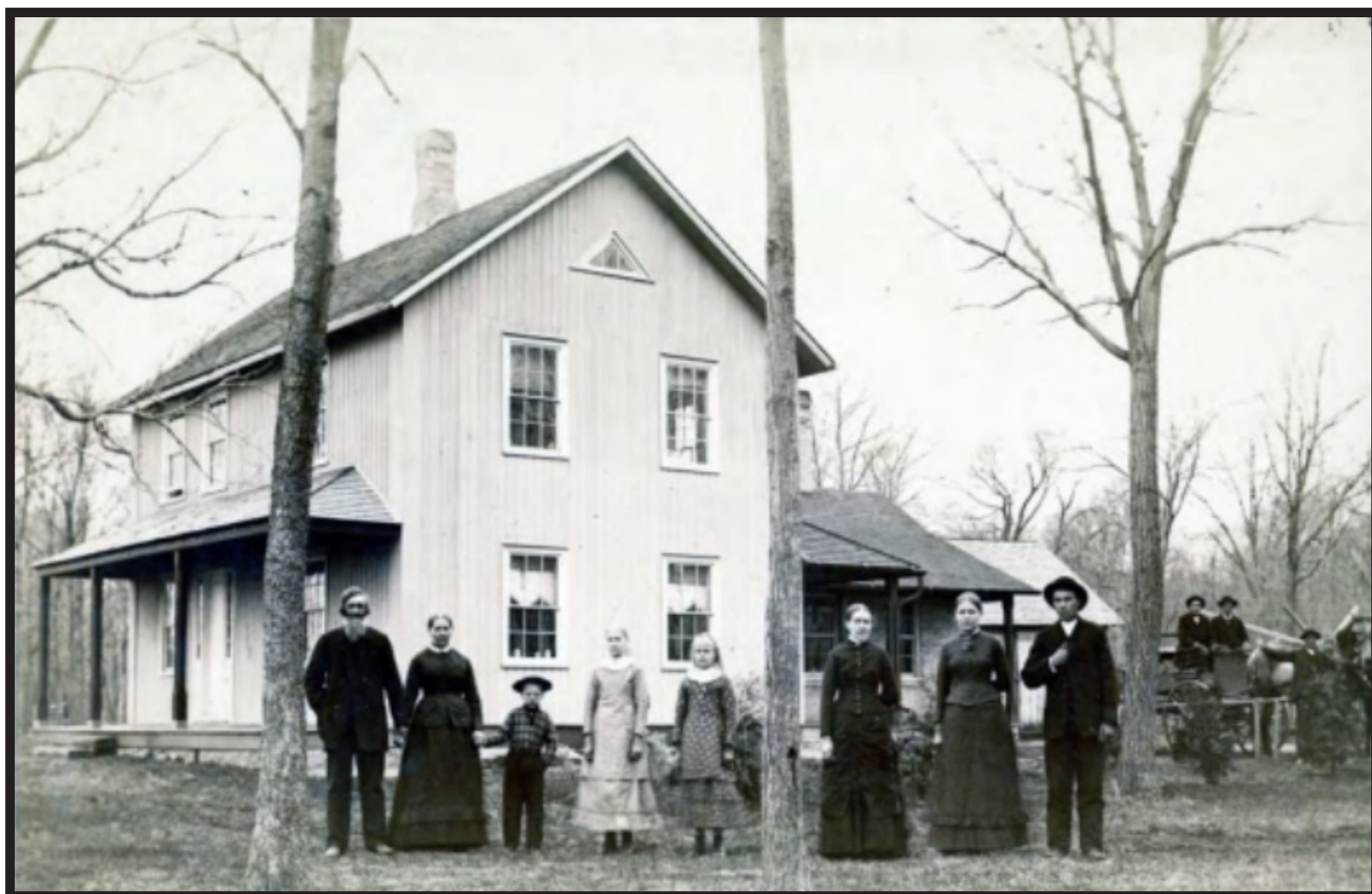
1885 Photograph of the Peterson Farmhouse.
