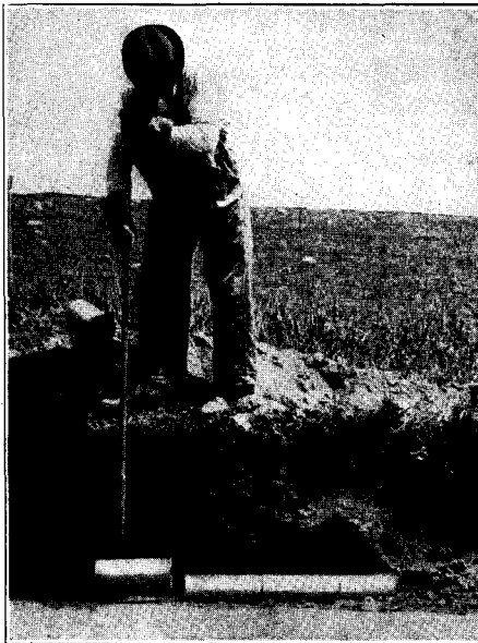
Fig. 34a. Laying Tile with Tile Hook— Sectional Side View
