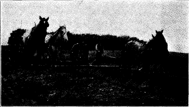
Fig. 43. Filling Trenches with Plow
