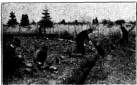
Making Junctions by Hand and Laying Tile
