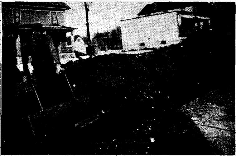
Fig. 44. Type of Scraper Well Adapted to Filling Trenches and Digging Shallow Ditches
