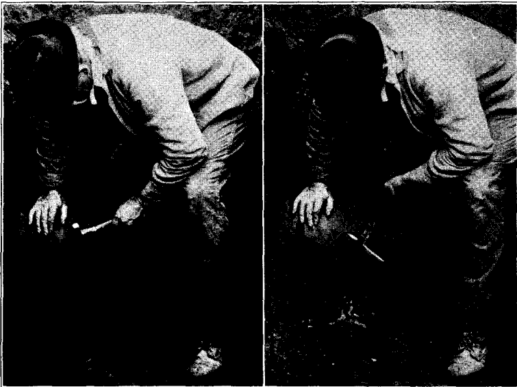
a. Starting the hole b. Enlarging the hole Fig. 38. Cutting a Hole for a Junction in a Large Main
