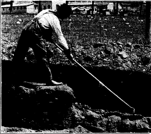
Fig. 25. Method of Finishing Tile Trench to Grade
