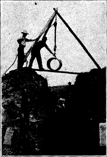
Fig. 36. Handling Large Tile with Derrick
