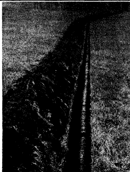
Fig. 34b. Line of Tile in Trench, Ready to Blind
