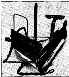
Fig. 4. Push Grader for Shallow Surface Ditching
