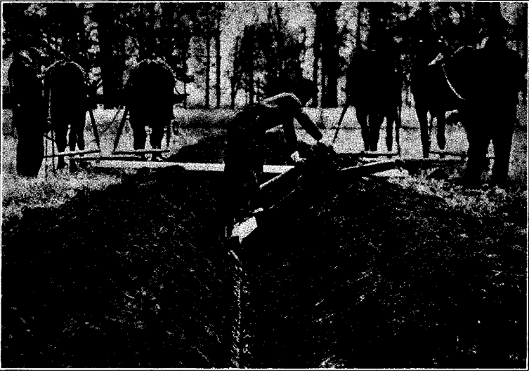
Fig. 5. Digging Flood Ditches with the Push Grader Shown in Figure 4.
