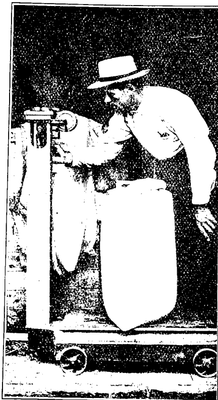
FIG. 3.—WEIGHING TO TEST THE OVERRUN OR UNDERRUN FROM A THRASHING MACHINE.
