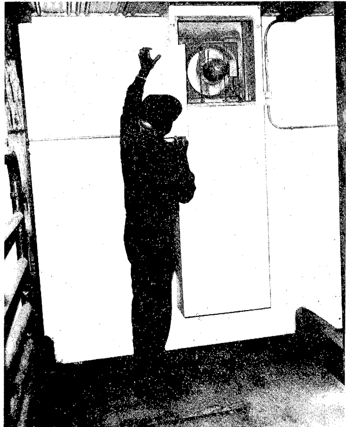
Figure 10. In winter, air near the floor in a livestock building can be as much as 10 degrees cooler than air near the ceiling. To conserve heat and energy, a duct as shown should always be used around the continuously operating exhaust fan or fans. An equal amount of moisture but less heat is removed than when air is exhausted from the ceiling, making a higher ventilation rate and thus greater dilution of contaminated barn air possible.
