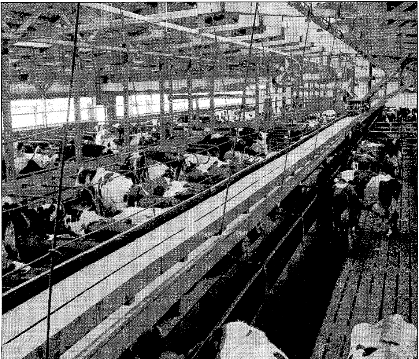
Figure 1. This naturally ventilated, slat-floor, free-stall dairy barn located in southern Minnesota is 80 x 200 feet and contains 206 stalls. There is a continuous, 16-inch-wide, uncovered open ridge at the roof peak together with 4-foot-high vertically operated wall vents. The ridge and vents run the full length of the building on both sides. Wall vents are manually controlled with winches. Cows are milked in a double-eight herringbone parlor (figure 8). There is a liquid manure tank 85 x 200 x 10 feet beneath the barn with storage capacity for about eight months.
