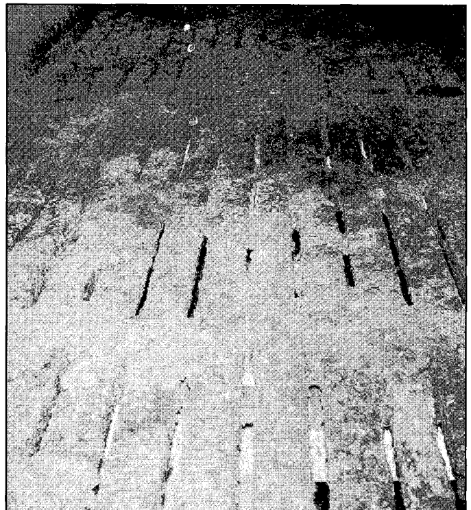
Figure 18. Typical slat-floor appearance in a cold, free-stall barn during winter. Frozen manure will quickly work through when weather moderates.
