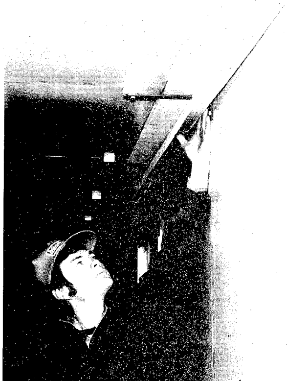
Figure 14. An adjustable slot inlet in the winter position. Picture was taken on a day when the outside temperature was -34^{\circ} F. Some condensation is evident, which is normal. In summer, the baffle is moved inward to the ceiling stops, enlarging the opening at the wall to 4 inches.
