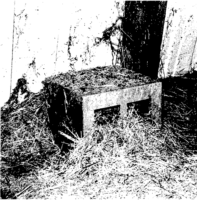
Figure 21. Air supply to ceiling intake in stable below must enter through this plugged opening in mow of two-story barn. Little air can pass through. Result, poor ventilation system performance.
