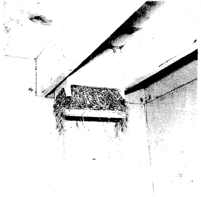
Figure 22. This ceiling intake through the ceiling of a two-story calf barn was deliberately plugged to "prevent draft." Result: faster air entry and more draft through remaining open intakes. Closing intakes will not solve a ventilation problem; it only makes matters worse. The underlying cause must be determined and corrected.
