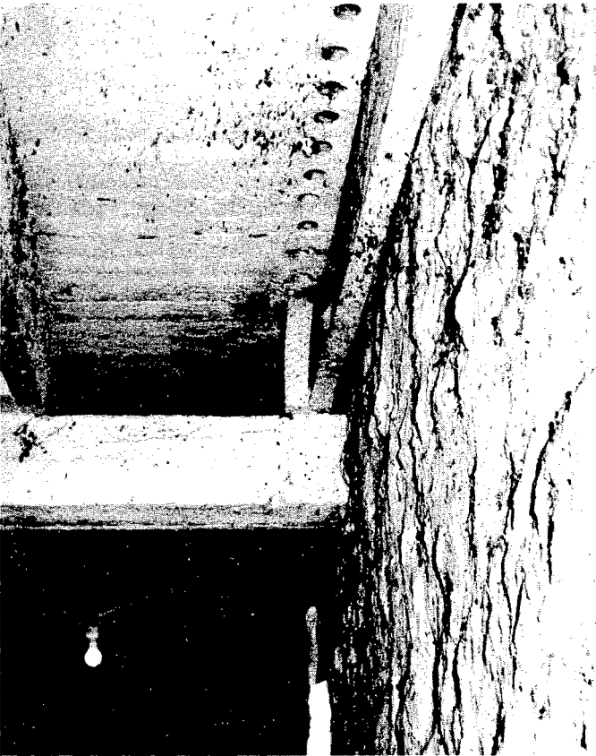
Figure 23. A satisfactory winter-air-intake system was made in this two-story barn by drilling 2-inch diameter holes about 10 inches on center through the mow floor to the space above.
