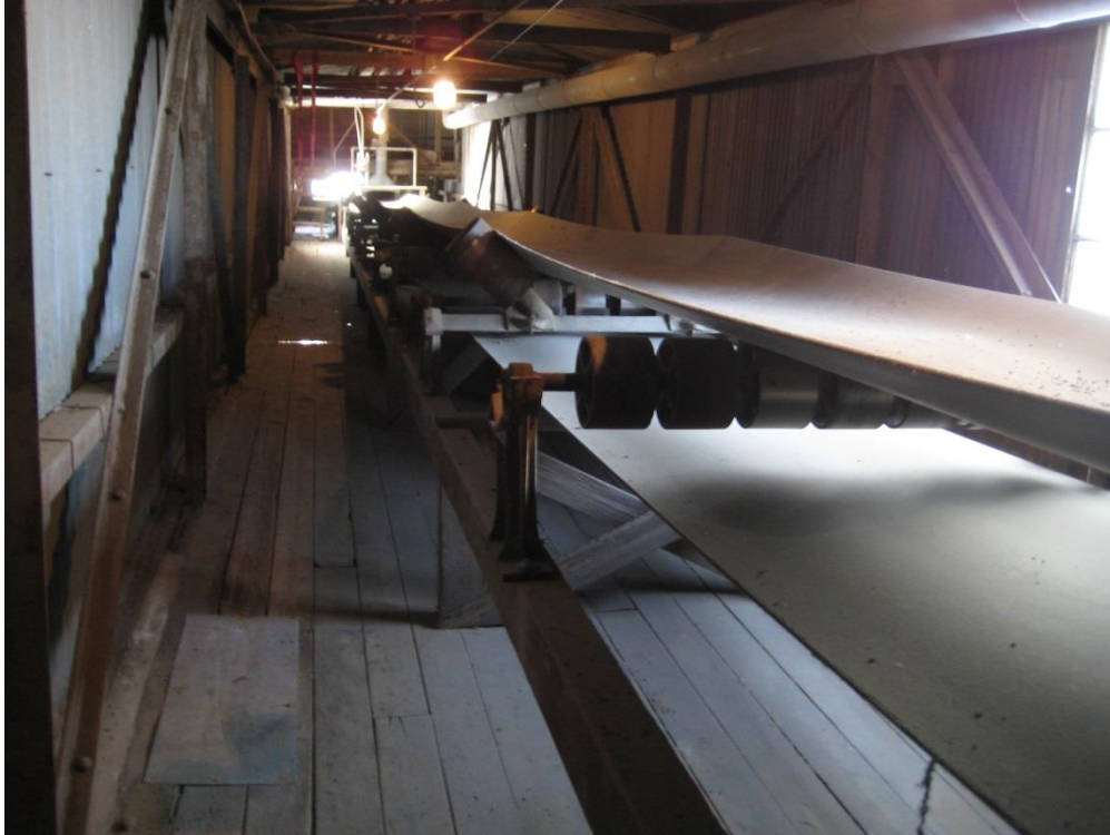
At the upper conveyor galleries connecting the circular storage bins the many safety hazards include floor hatches -- now secured -- which lead to 100-foot drops to the ground.
