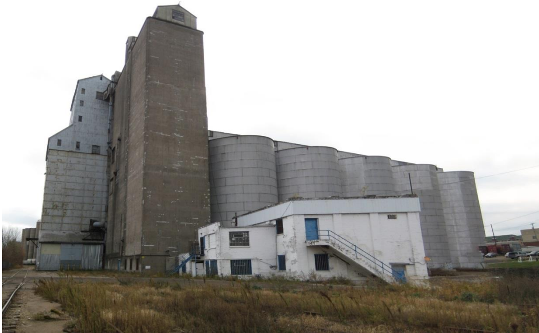
View from the west showing, from left to right, the original 1901 steel head house, the 1938 concrete head house and the 60-foot tall steel grain bins. In the foreground is the office, machine shop and garage.
