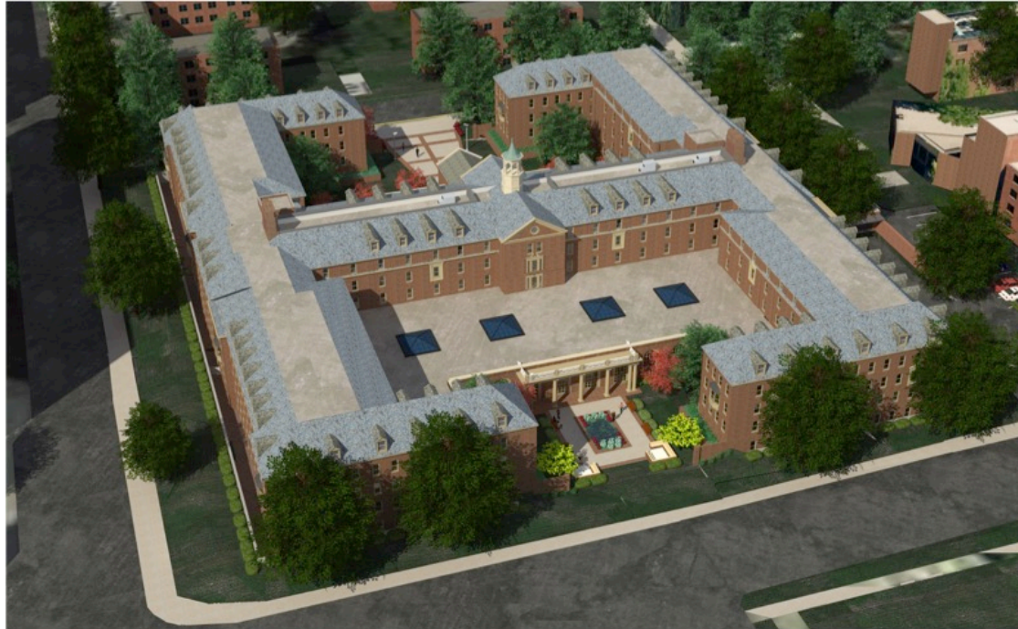
Aerial View from the Southwest
