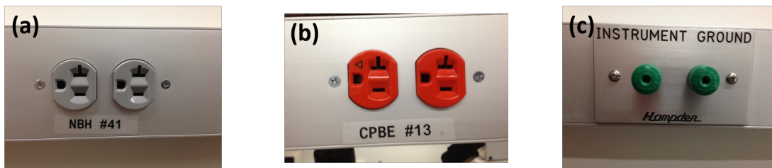
Figure 3.7: The three types of grounding receptacles available in the lab. The dirty ground shown in (a) is used for all equipment not in direct electrical contact with the sample, so as to protect the sample from surges on the line and to avoid contaminating the noise floor. The orange or “clean” ground shown in (b) is used only to ground the experimenter in this work, as its isolation from dirty ground is not sufficient for other uses. All equipment involved in direct measurement of voltages in the experiment is connected to the instrument ground in (c). Instrument ground is also used to ground the sample itself to protect from transients, which can cause sample failure.
