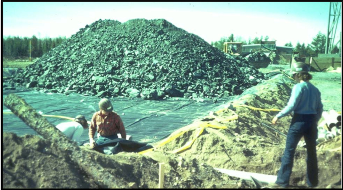
Figure 1-6. Photograph showing the construction of large-scale AMAX test piles (from Lapakko et al., 2004).
