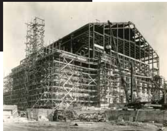
Northrop under construction in 1928
