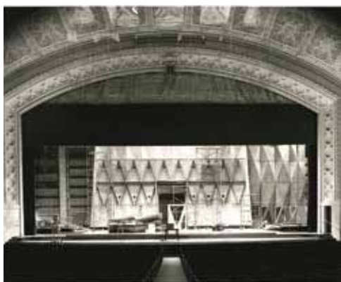
This steel acoustic shell, installed in 1961, was the first of its kind in the world.
