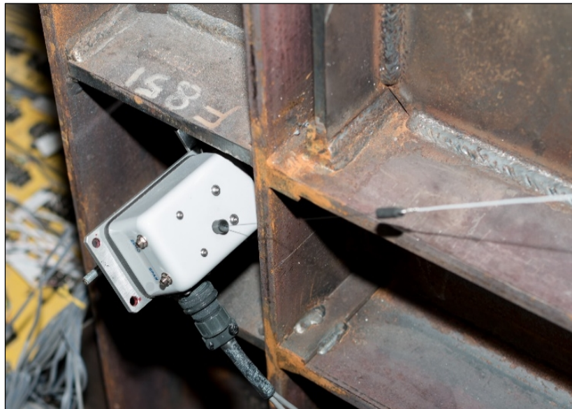
Figure 4-13: Diagonal string-pot installed on frame
