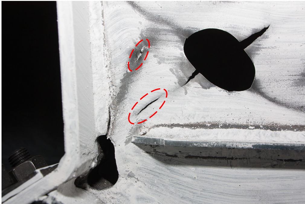
Figure 5-20: Damage in the LM subpanel during the last cycle of test 4 (t=36.75)
