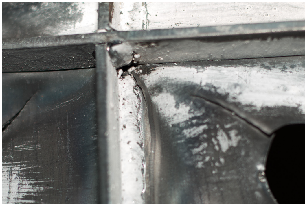
Figure 5-16: Test 3 – Cracking at stiffener weld termination
