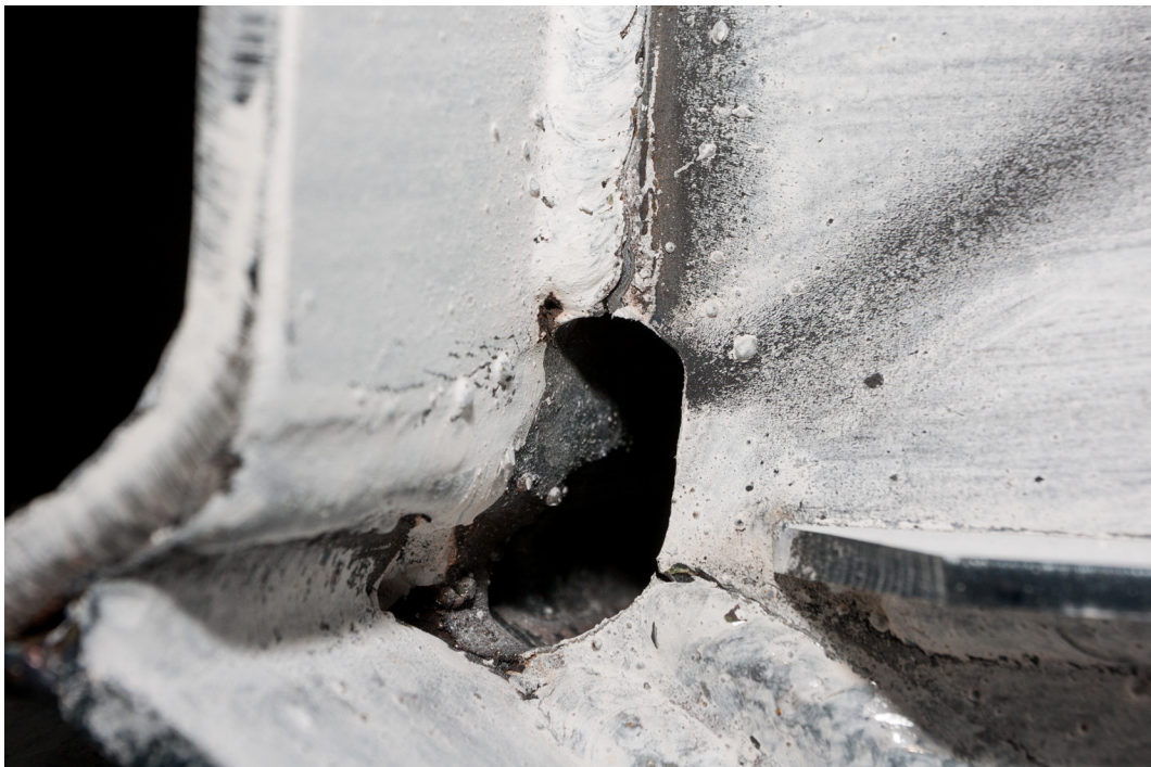
Figure 5-32: Cracks at welds termination (t=24.50)
