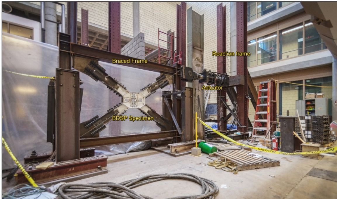
Figure 4-1: T. Galambos Structural Engineering Laboratory with first BDSP specimen
