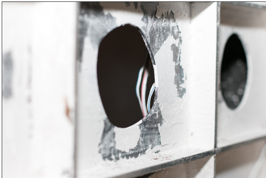
Figure 5-7: Test 2 – Out-of-plane displacements in CM subpanel
