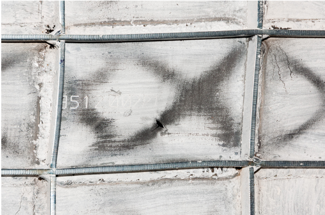
Figure 5-31: First crack in CM subpanel, test 6 (t=27.50)
