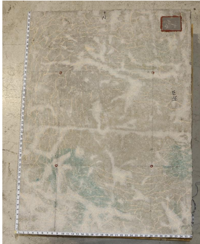
Figure 34. Photograph of condition of slab D.
