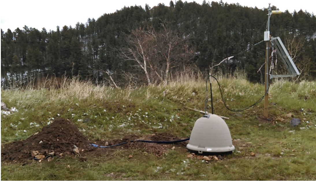
Figure 6.6: Full RRDG station, including the sealed seismometer vault (under dirt pile), electronics doghouse (beige igloo near center), solar panels (middle right, attached to center of wooden post), GPS antenna (on top of wooden post), and radio antenna (green cylinder just below GPS antenna).
