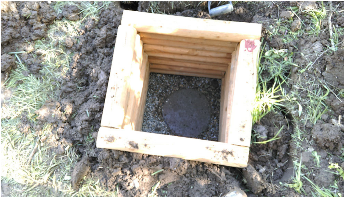
Figure 6.4: Seismometer vault enclosure at DEAD surface station. The timber enclosure and the concrete cylinder are shown, but the layer of foam board insulation is not pictured.
