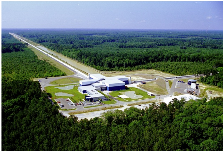
Figure 2.1: Aerial view of the LIGO observatories at Hanford, WA (top) and Livingston, LA (bottom). The laser and main optics are contained in the large buildings at the vertex of the two beam tubes. Figure reproduced from Ref. [1]. Copyright IOP Publishing. Reproduced with permission. All rights reserved.
