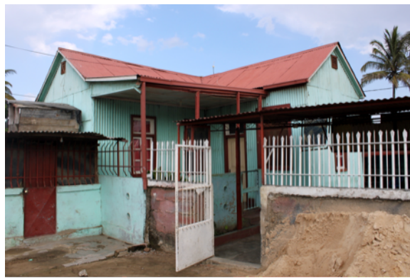
Fig. 1.3. An L-plan wood-and-zinc house built by Jochua Guambe in the 1930s. Note the small pigeon coop above the storage room on the left. (Photo: the author)
