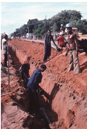
Fig. 5.15. Volunteers dig trenches for water pipes, 1978. (Source: Ingemar Sävfors)
