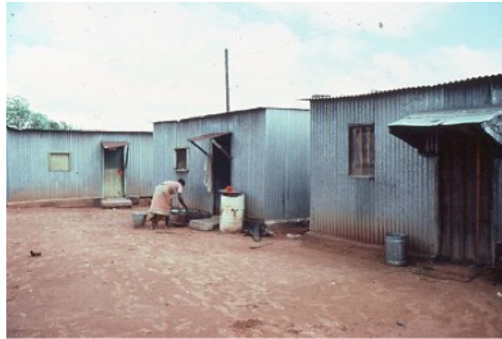
Fig. 1.2. Conventional wood-and-zinc houses, mid-1970s. (Source: Ingemar Sävfors)
