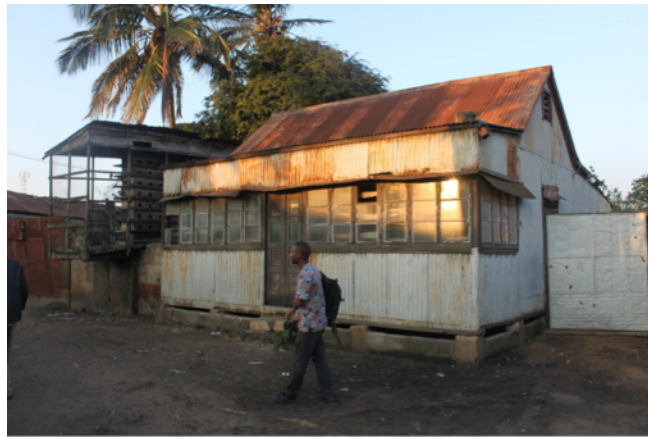
Fig. 1.8. The Araújo residence, built in the 1920s by a Goan railroad employee. Partially visible to the left of the enormous pigeon coop is the enormous componde built by António Araújo in the 1960s. (Photo: the author)
