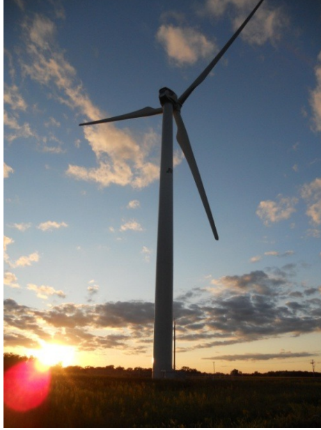
Figure 2.1: 2.5 MW Clipper research turbine located at UMore Park, Rosemount, MN.
