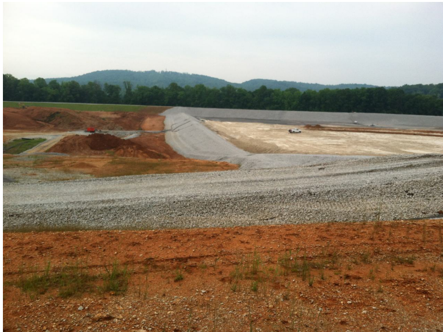
Figure 7: New gypsum ponds for scrubber waste
