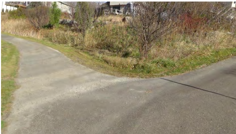
Photo 1. Sediment from the uphill residential area can be seen along the paved trail. The runoff travels from uphill, over the trails, and into the managed turf area on the left.
