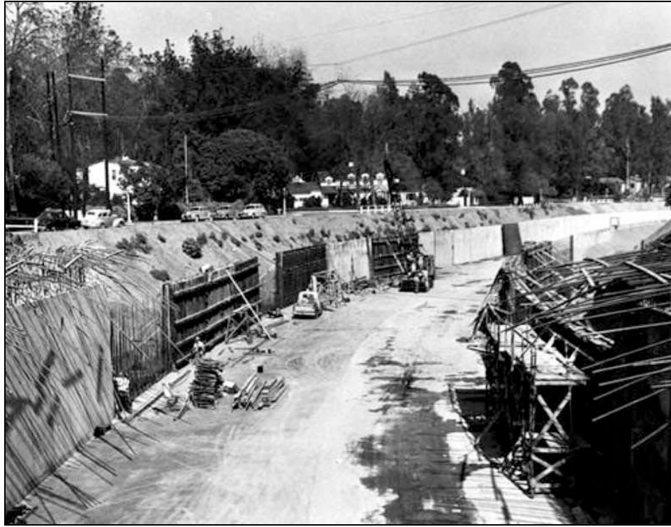
Figure 4.13. The concreting of the Tujunga Wash in Van Nuys, c.1967.
