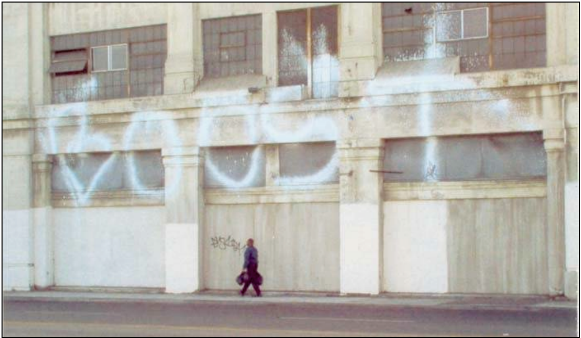
Figure 3.28. A fire extinguisher “Boost” tag on a Downtown factory, c. 2000. Source: www.50mmlosnagels.com
