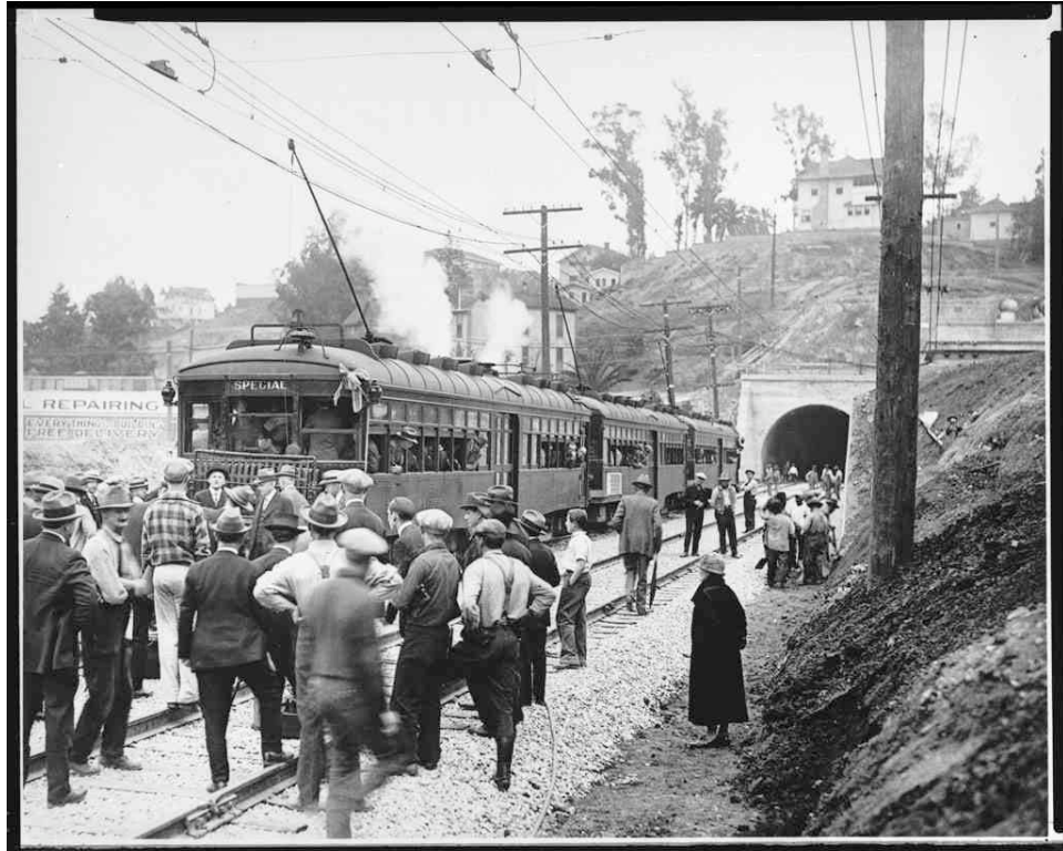
Figure 5.3. Opening of the Belmont Tunnel at the Toluca Station, 1928. The tunnel is visible in the background. California Historical Society Collection, 1860-1960, USC Digital Archives.
