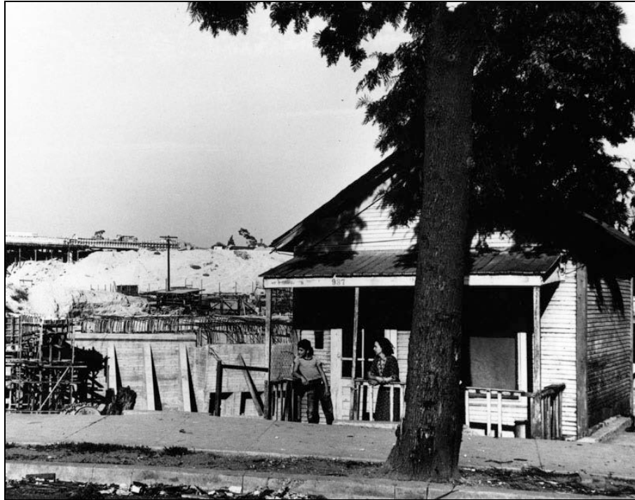
Figure 4.25. “Demolition work in preparation for the construction of the Harbor Freeway near Court Street.” A Harbor Freeway overpass is visible at the left of the image. Photo by Leonard Nadel. Los Angeles Public Library Photo Collection.
