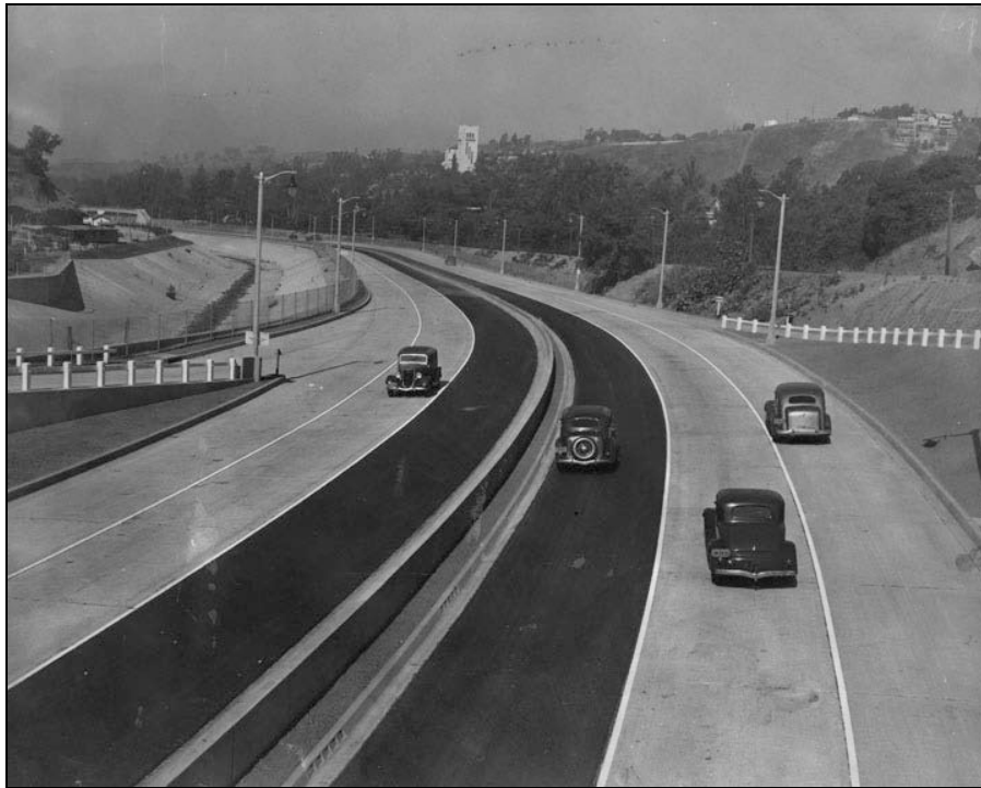
Figure 4.9. “First motorists to travel over the new link at 53 rd Street,” 1940. The concreted arroyo is visible at left. Herald-Examiner Collection / LAPL
