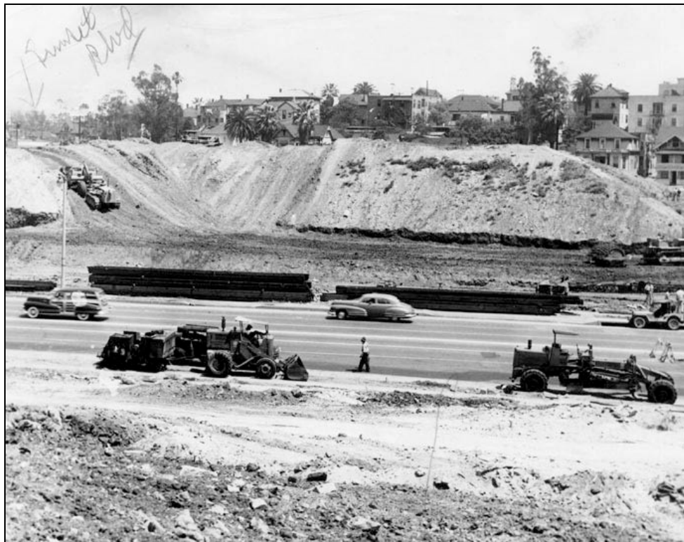
Figure 4.2. Sunset Boulevard under construction, c. 1936. LAPL Photo Collection.
