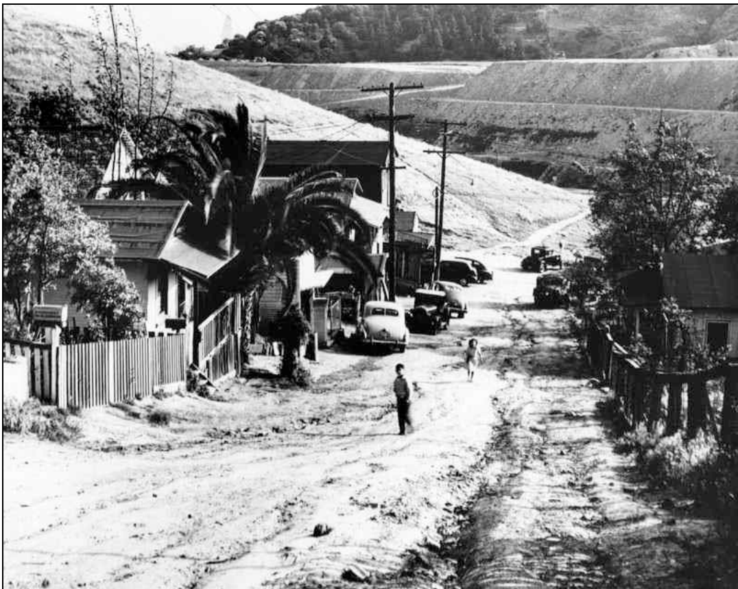
Figure 4.36. Two children on an unpaved road in Chavez Ravine, 1950 The faint outline of City Hall in the distance. Photo by Leonard Nadel. L.A. Public Library Photo Collection.
