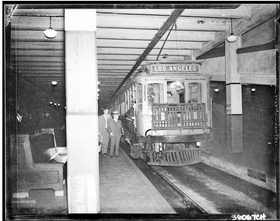
Figure 5.4. Hollywood Subway, 1930. Chamber of Commerce Collection, USC Digital Archives.
