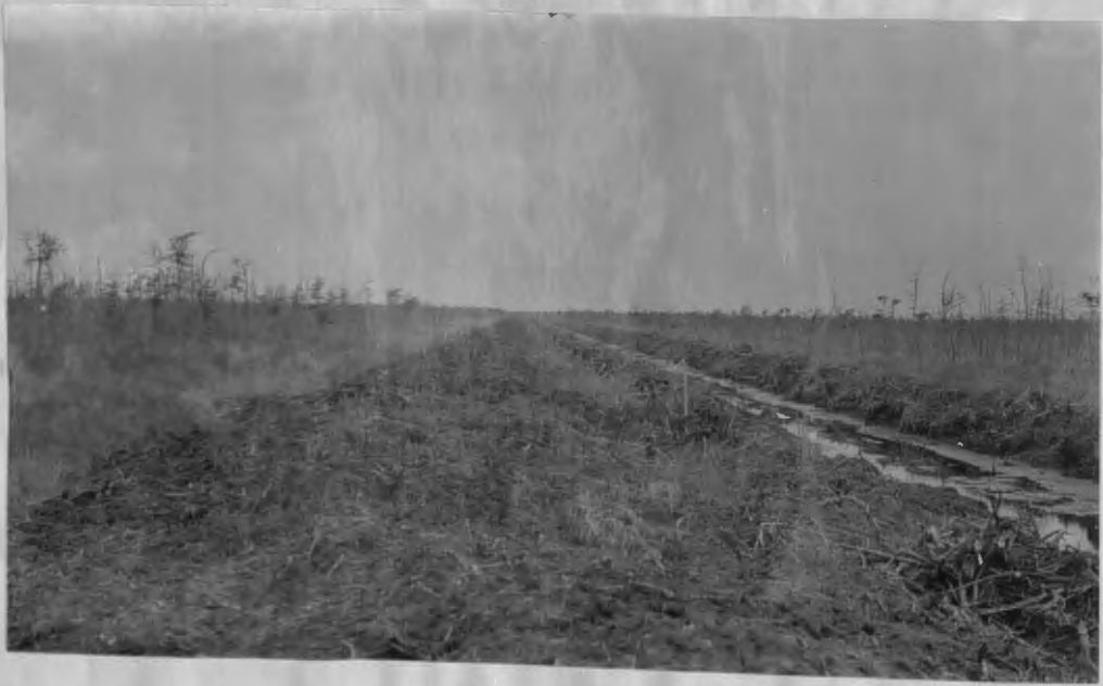
A recently constructed ditch through the low timber type of peat at Dibbell, showing the small size of the roots and stumps buried beneath the surface.
