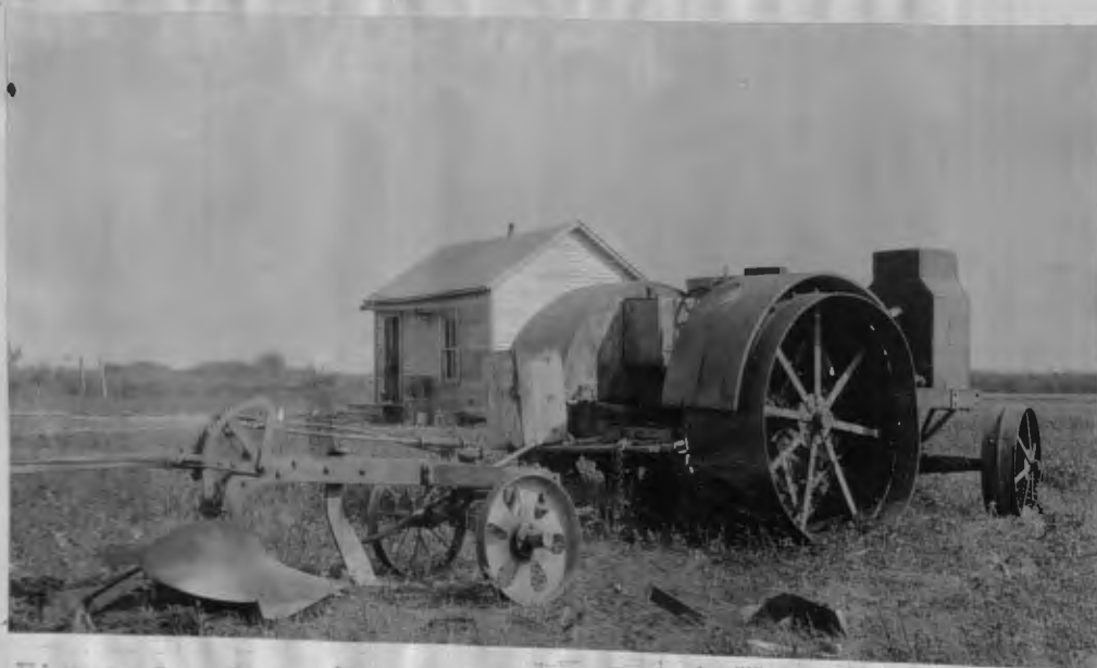
Figure 1 - Deep (24-inch) traction-drawn plow, used on peat soils in Pennington County.
