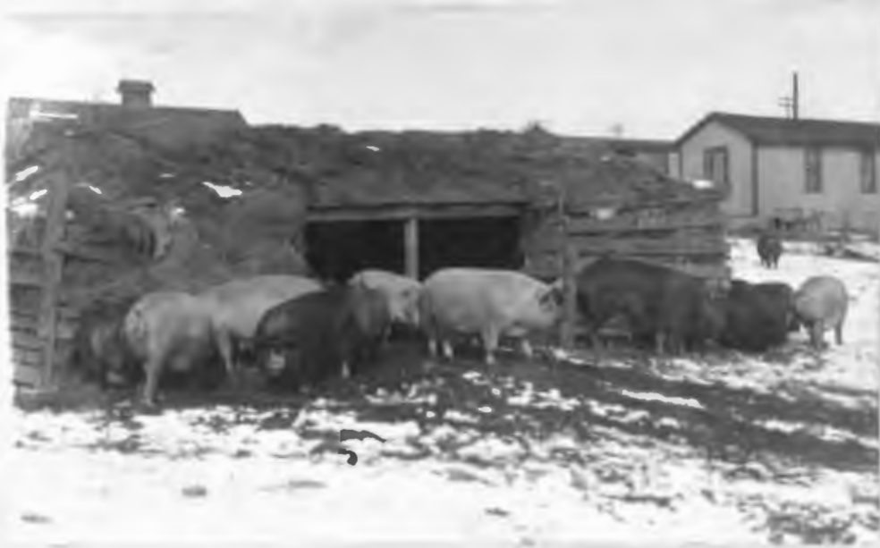
Figure 11 - An easily constructed home-made hog shelter that answers the purpose
