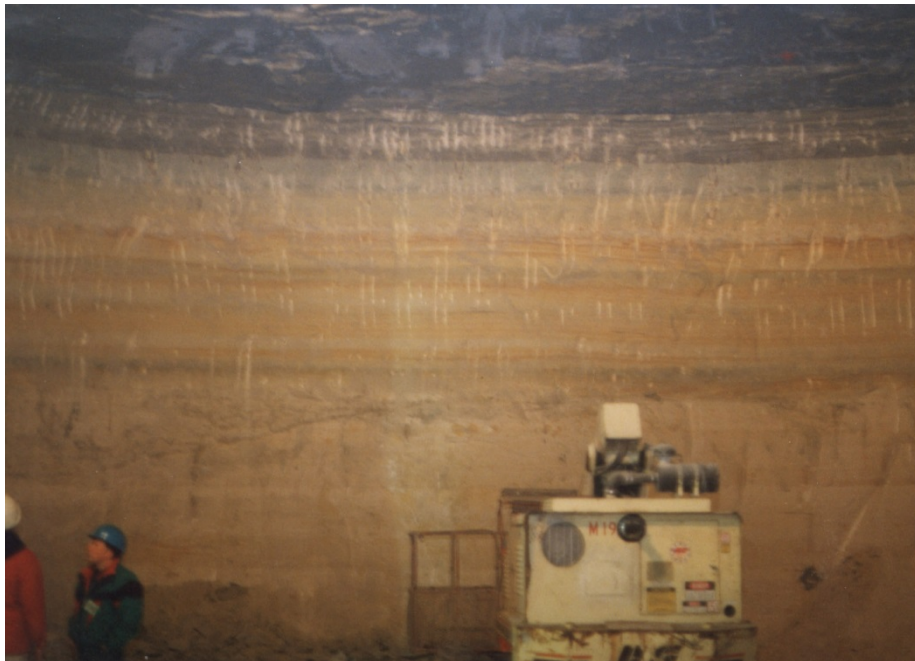
Figure 2-6: The north wall of cavern 1 showing a horizontal seam in the St. Peter sandstone.
