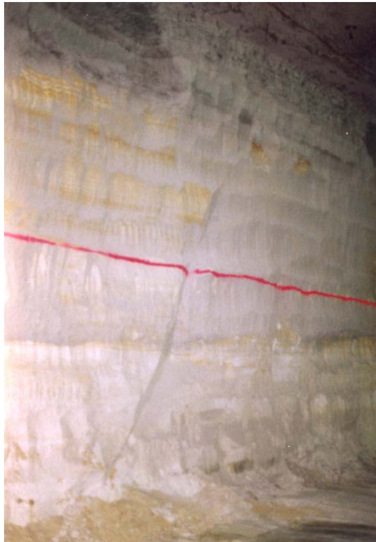
Figure 2-7: View of west wall of cavern 1 showing vertical jointing in the St. Peter sandstone.
