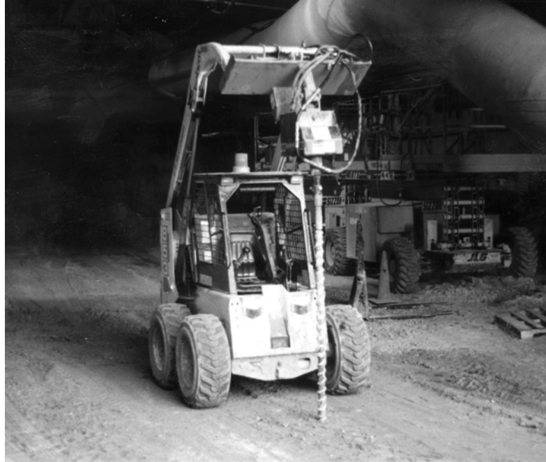
Figure 5-8: 753 Bobcat skid loader and drill attachments for drilling boreholes for pressuremeter testing.
