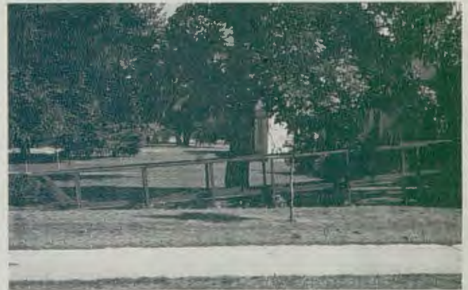
The home of Mr. and Mrs. Edmund Fuller of St. Paul has the advantage of a large front yard, making a long ramp possible. The longer the ramp, the more gradual the slope can be.
