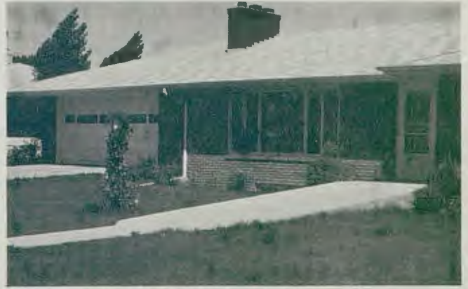
This ramp at the home of Mr. and Mrs. Gordon C. Green of St. Paul starts with a concrete slab that is level with the entrance sill. The slope begins about 4 feet from the doorway.
