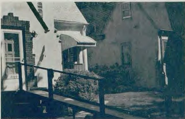
Mr. and Mrs. Arthur Ahlgren of Minneapolis built their home before a ramp was needed. Although the ramp covers the front steps, walking up the ramp is made safe with a strong railing and use of paint containing a nonslip material.
