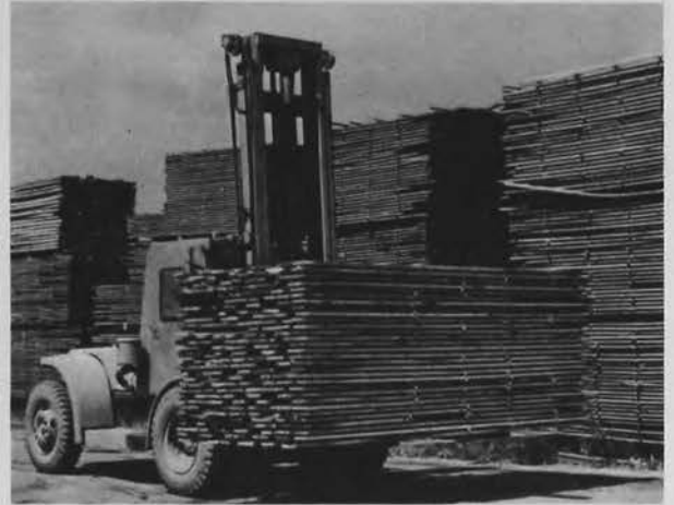
Figure 3.—Stacking stickered package of lumber.
