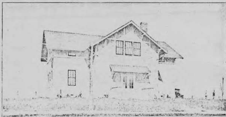
Fig. 1. Institute Hall, as Rebuilt in 1921
