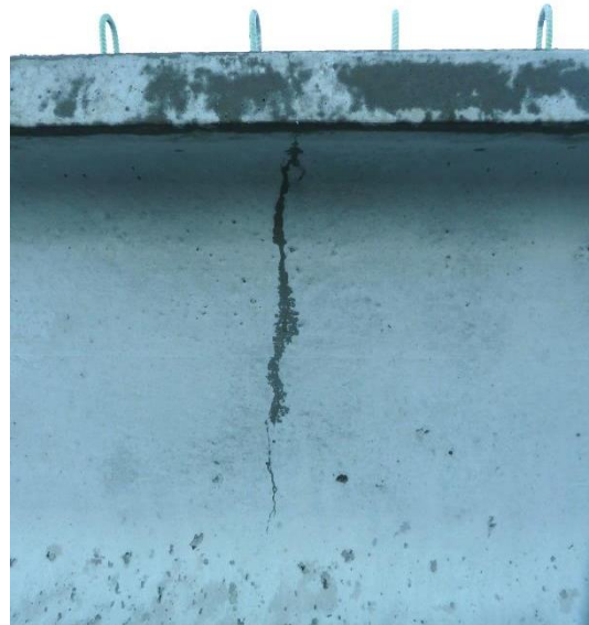
Figure 6.26: Observed concrete cracking near hold-down just before release during Test 1
