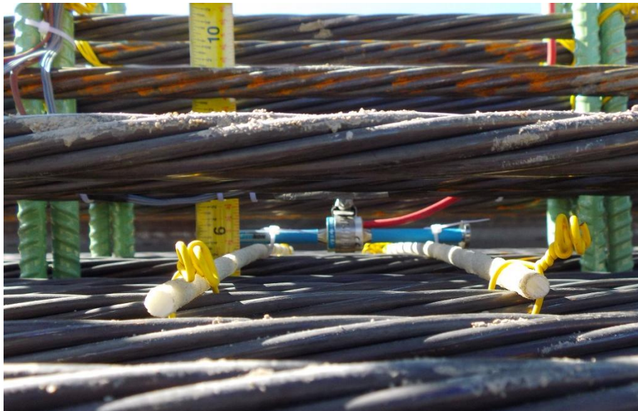
Figure 6.1: Vibrating wire strain gage near the center of gravity of the strands at midspan
