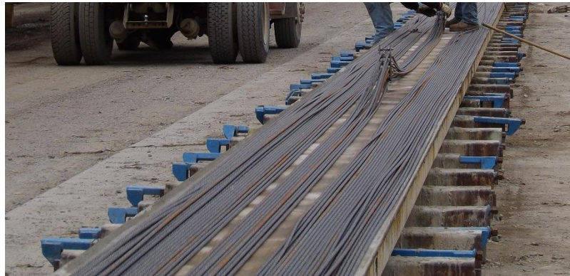
Figure B.1: Strands lying on precasting bed near hold-down prior to tensioning
