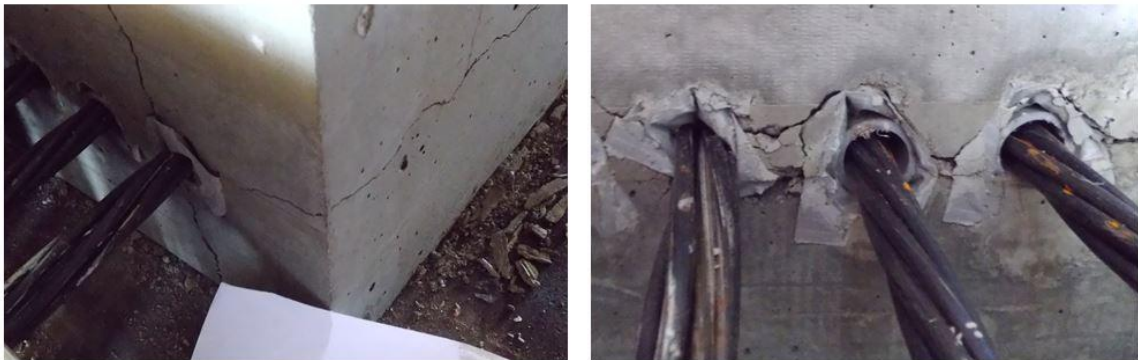
Figure 5.19: Girder 3 cracks; Crack 1 (left) and Crack 2 (right)
